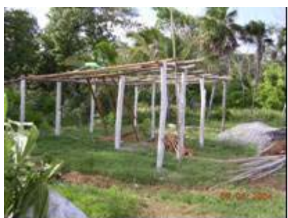
New Construction for the gathering of separated material
