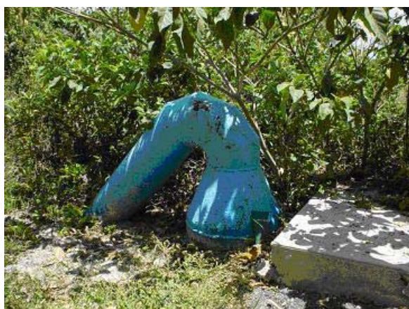
Figure C-5: Injection Well of CAPA in Othon P. Blanco
