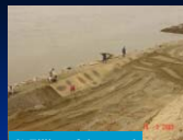
3) Filling of river sand below El. 161.5m
