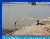
8-2) Putting rubble stones on mattress by backhoe
