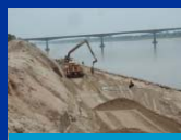
5) Spreading and compaction by Bulldozer above El. 161.5m
