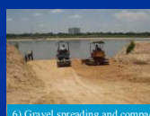
6) Gravel spreading and compaction for the restoration at temporary access road
