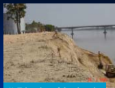
1) Trimming of the slope by backhoe
