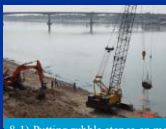
8-1) Putting rubble stones on mattress by wire straw-basket
