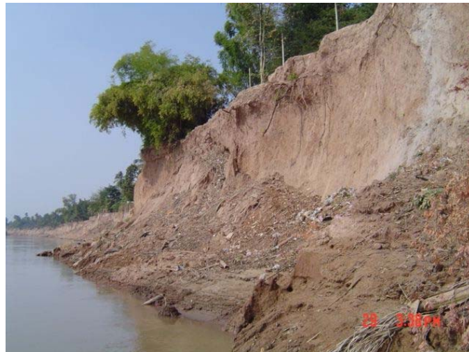
Figure 4.8 Typical Riverbank at Ban Hom Site
