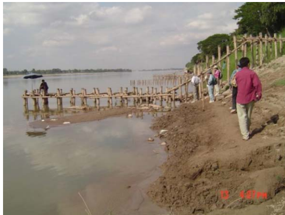
Figure 1.7 Sedimentation between Wooden Pile Dike Groyne Works
