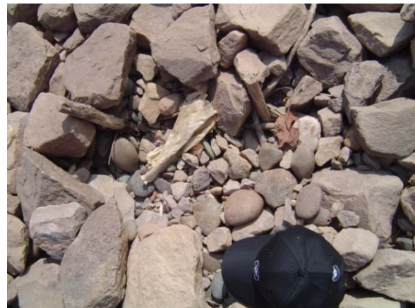
Figure 1.12 Sediment Material under the Slope Covering Riprap at Sibounheuang Site
