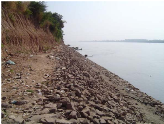
Figure 1.11 Downstream View at Sibounheuang Site
