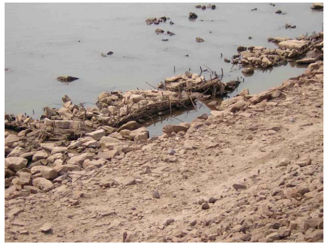
Figure 1.4 Ripraps on SODA Mattress Work
