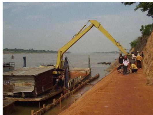
6) Check of the compaction and finishing of the embankment level
