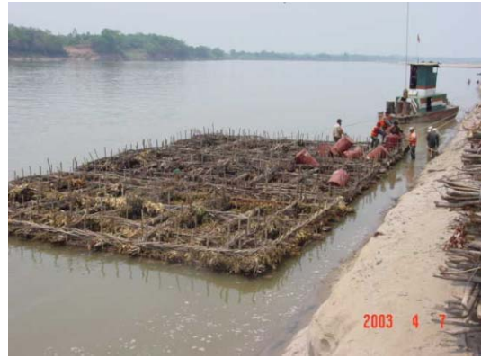
2) Placing floating Soda mattress at the planned position by boat
