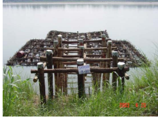
2) Placing Soda mattress at the planned position by boat and manpower
