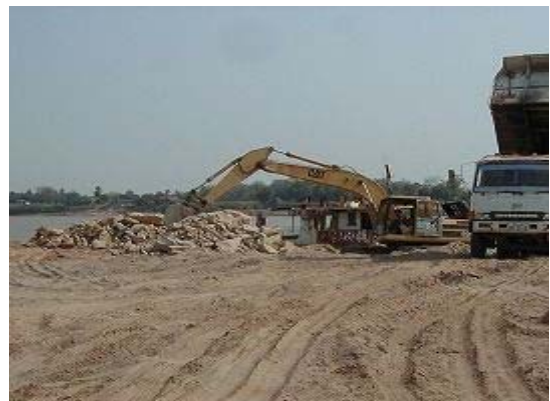
6) Loading into Barge
