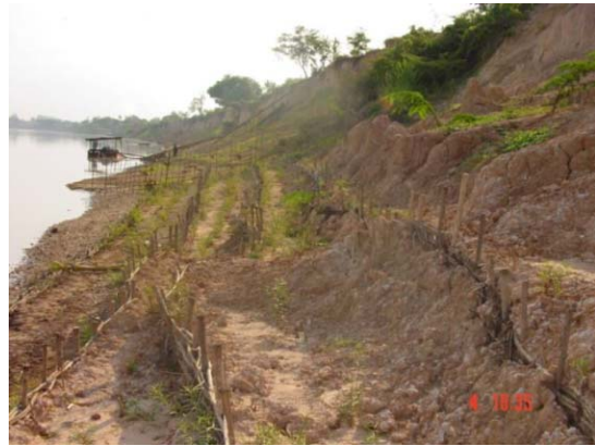
Completed Soda-net Works (Down stream Side)
