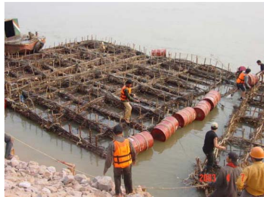
4) Connecting Soda mattresses by manpower
