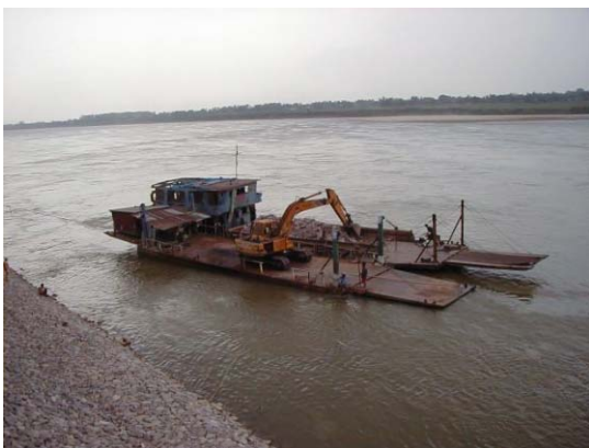
5) Stone placing on Soda mattress from barge
