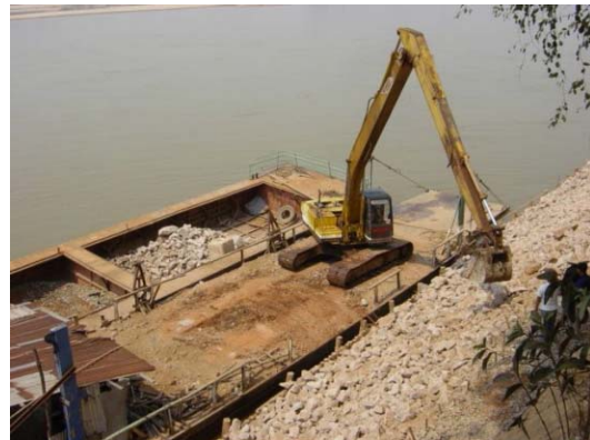
4) Cobble placing by backhoe on barge
