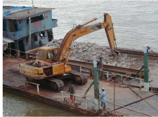
2) Stone transported from Kao Liao stockyard by barge and loaded by backhoe
