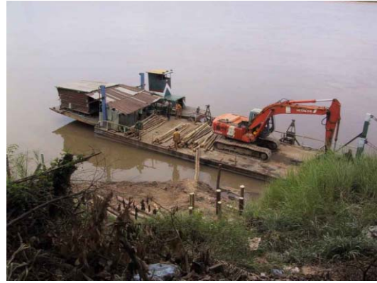
2) Transporting to the wooden piles to the planed location by barge
