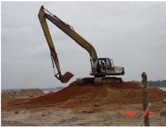
3) Laterite loading by backhoe
