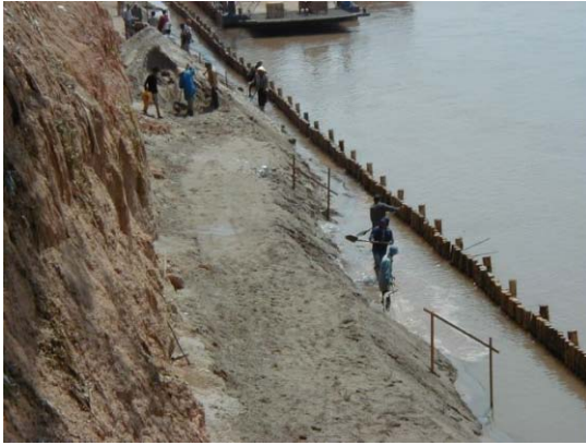
1) River sand filling and moisture arrangement
