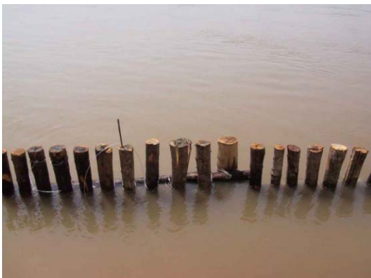
5) Close view of pile arrangement
