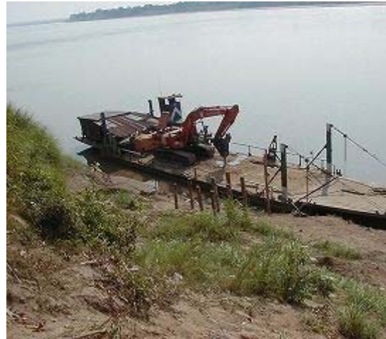
2) Barge and piling
