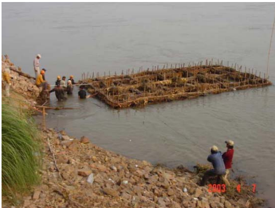
3) Making fine adjustment by manpower
