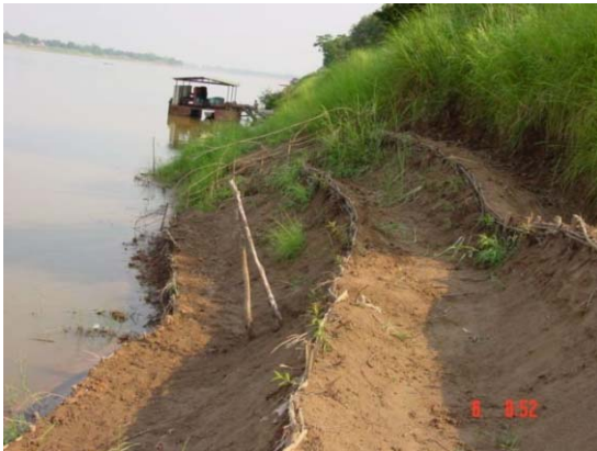
Completed Soda-net Works
