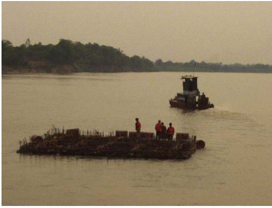
1) Towing floating Soda mattress by boat from Kao Liao stockyard into the site
