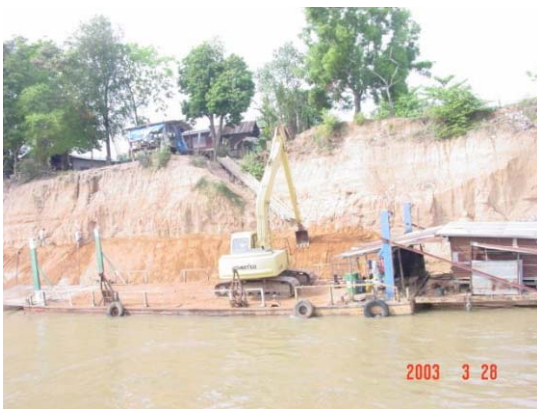
5) Filling and slope compaction by backhoe on barge
