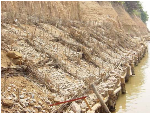
3) Condition of sand and gravel placing in the frame ( Taisya hurdle)
