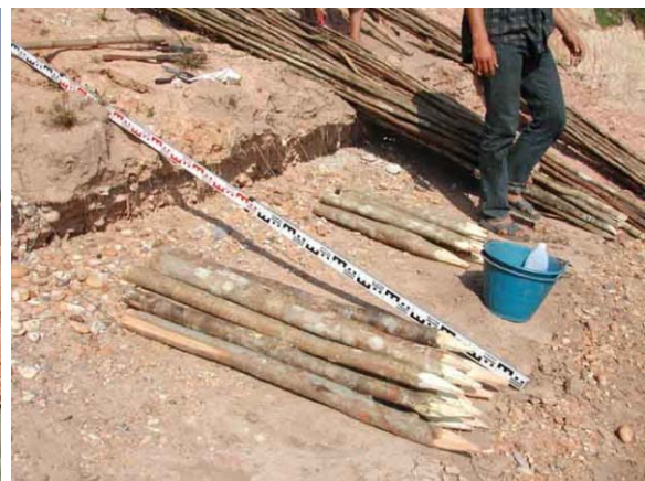
Short piles Length=0.7m, 0.9-1.2m \phi 5cm
