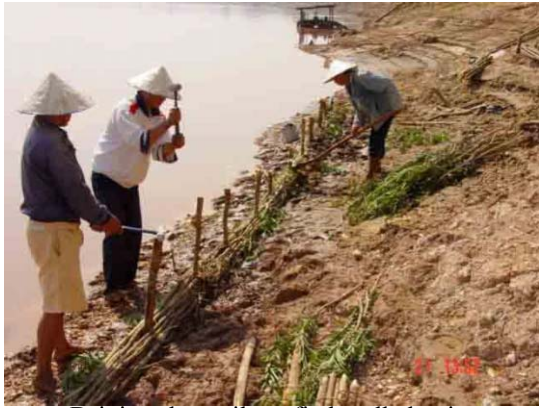
Driving short pile to fix bundled twigs
