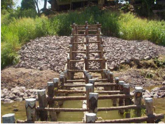
7) Riprap on the slope around connecting piles
