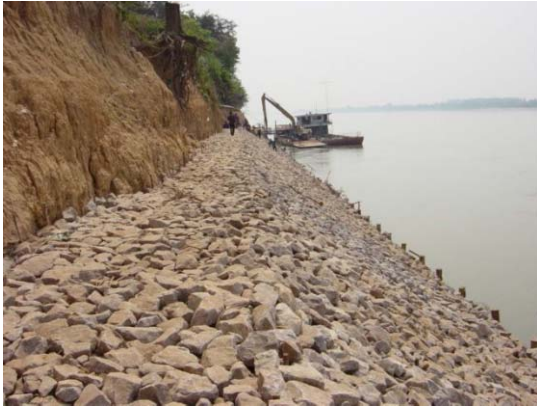
1) View of completed slope protection work
