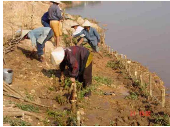
Situation of Making Soda-net Planting willow deeply
