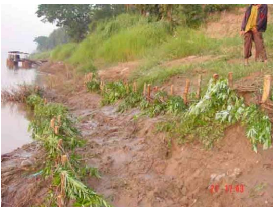
Situation of planted willow connected Soda-net
