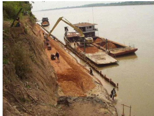
4) Compaction by vibration rollers and slope compaction by a backhoe
