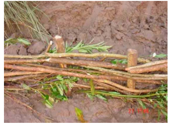
Planting willow connecting twigs and short piles
