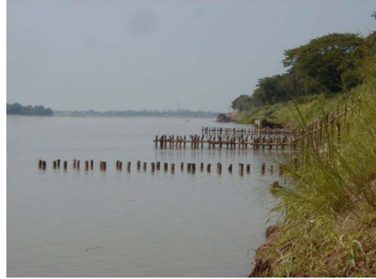
8) View of completed groyne works
