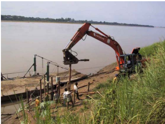
3) Piling work by backhoe (pushing down)
