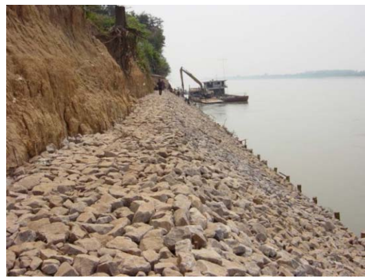
6) Completed cobble stone with willow branch works
