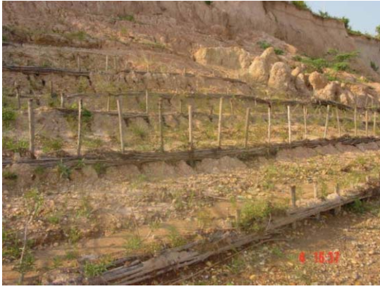
Completed Bundled tree works (Up stream Side)
