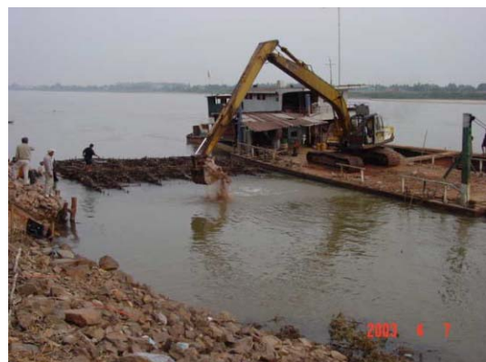
6) Putting rubble stones on mattress by backhoe on barge to submerge mattress
