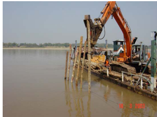
4) Piling work by backhoe with attachment to vibrate and hit a wooden log
