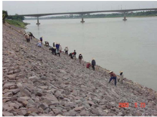
4) Stone arrangement by manpower
