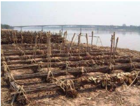
3) Soda Mattress under assembling
