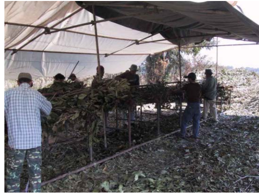
2) Making 'Rensai' (connection beam made of fascine)
