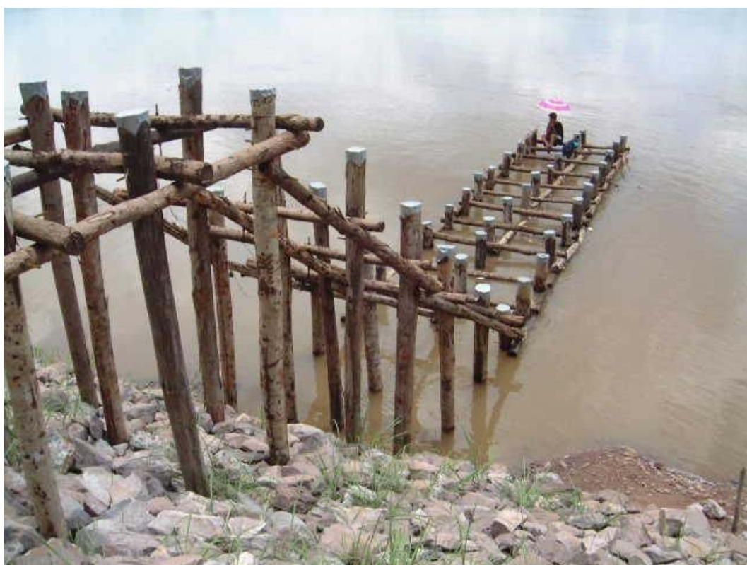
Wooden Pile Groyne and Riprap on Slope
