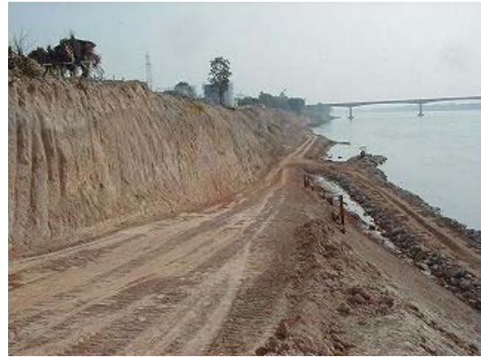
2) Temporary road near riverbed
