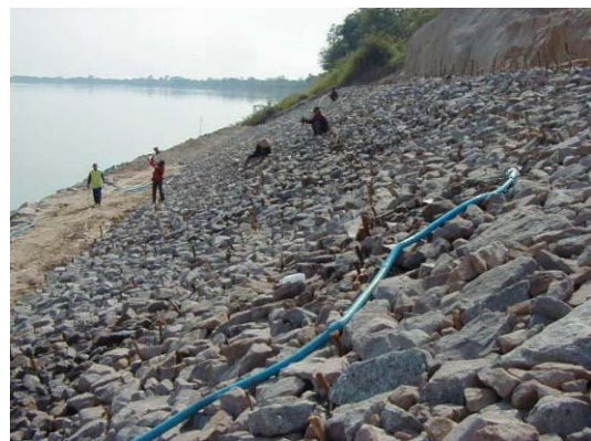
6) Finishing work of slope: Adjusting cobble placing
