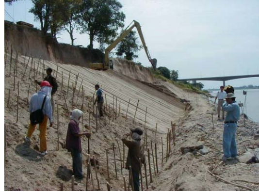
2) Compaction of slope and Kogui piling
