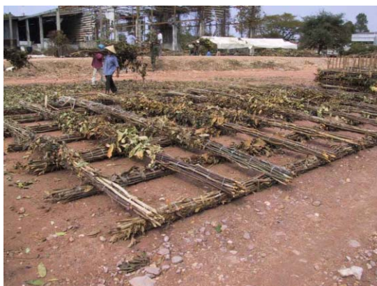
5) Arrangement of lower lattice structure by using 'Rensai'.
