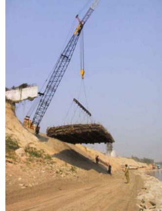
2) Lowering Soda mattress to the bank slope
