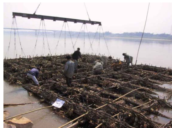
6) Connection of Soda mattress with up-stream one
