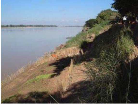
December 20, 2001 <Upstream Side>
