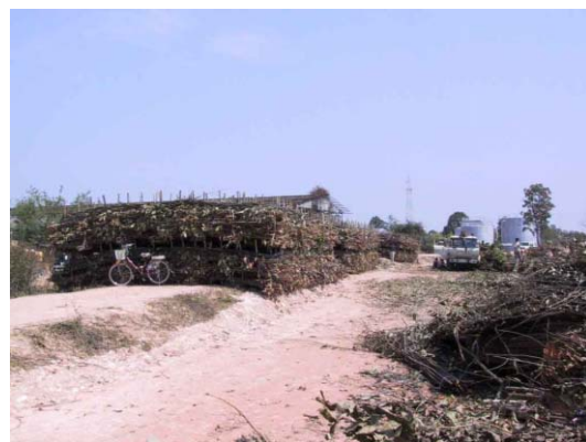
12) Piling-up of completed Soda mattresses
