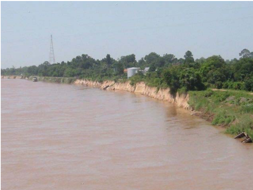
Before Construction (October 2002)
