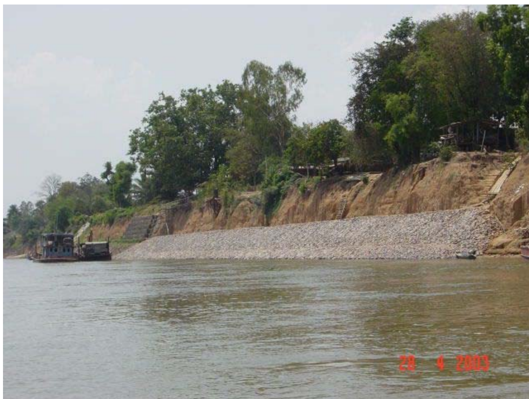
After Construction (May 2003)
