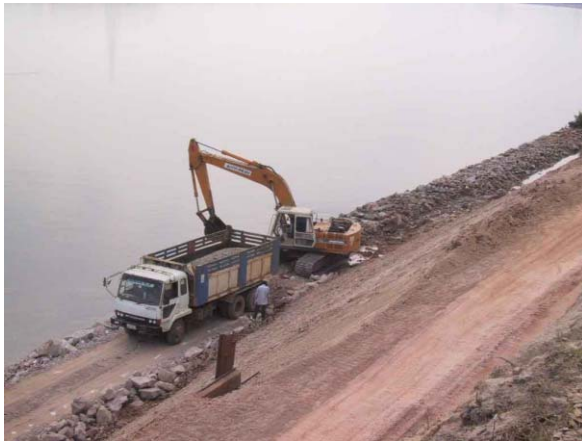
3) Supplying stones by Dump Truck
