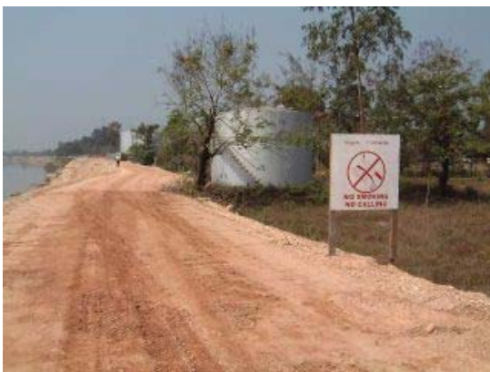
5) Situation along oil stockpiling
