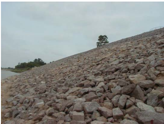
5) Completed stone covering slope
