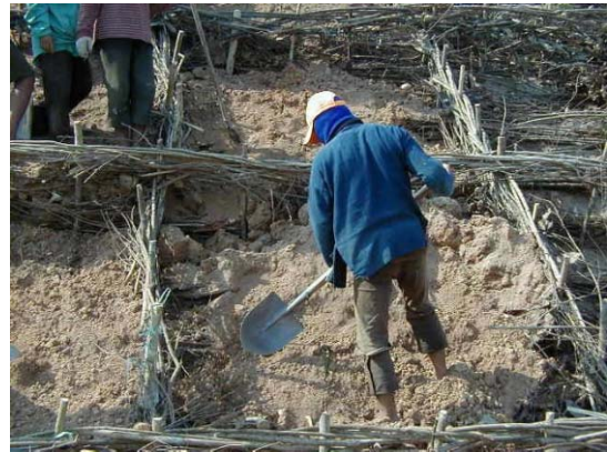
4) Sand and gravel placing in Taisya hurdle (T=20cm)
