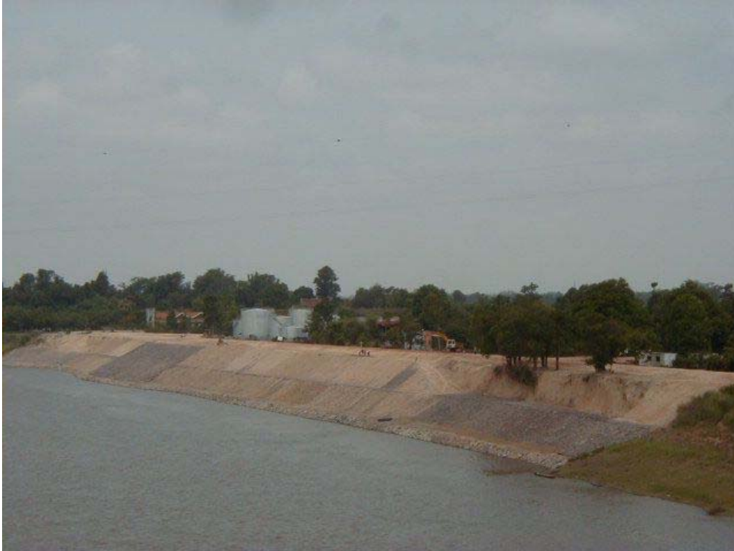
After Construction (May 2003)
