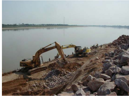
2) Stone loading by backhoe on the cat-walk level (El 161.5 m) of the lower slope
