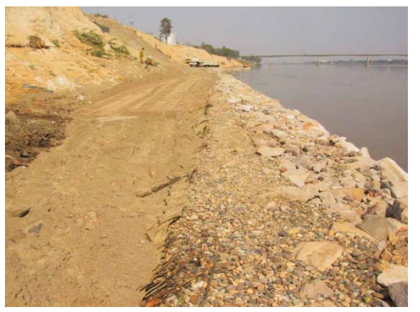
6) Placing bamboo net and sand behind gravel layer
