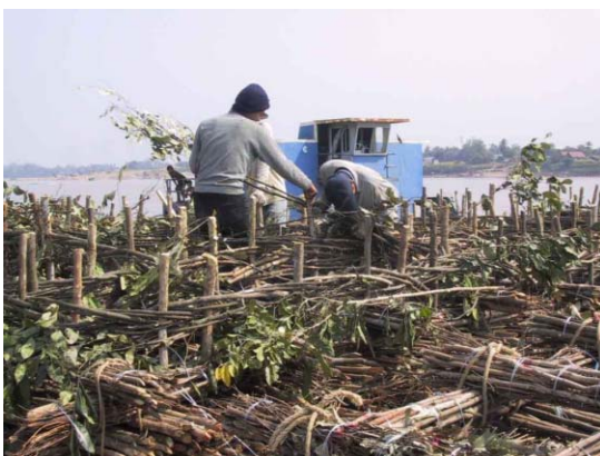
11) Hurdling work by using 'Taisha'
