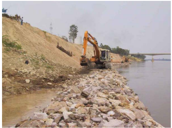
4) Placing crushed stone
