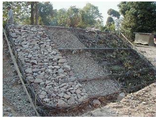
4) Model of Cobble Stone with Willow Branch Work demonstrated by the Study Team
