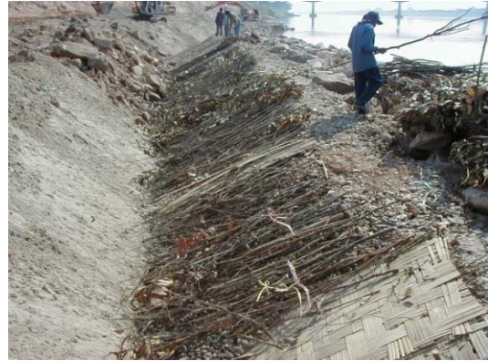
2) Tate-soda and bamboo net setting
