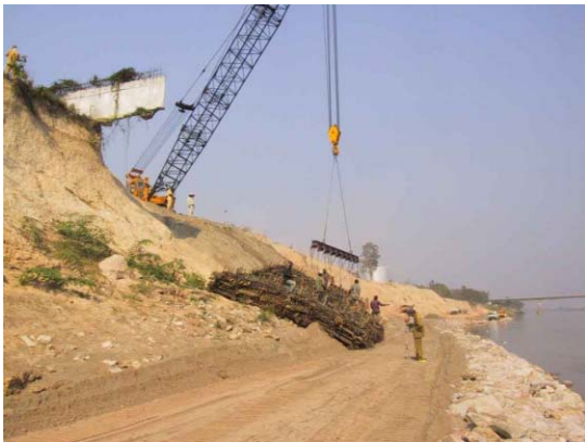
3) Temporarily placing for final setting
