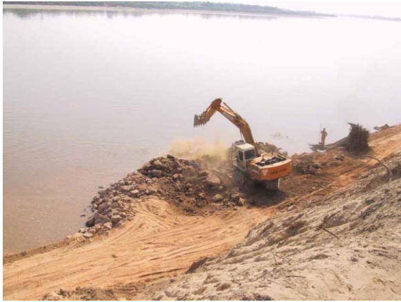
1) Starting filling stones for the foundation work
