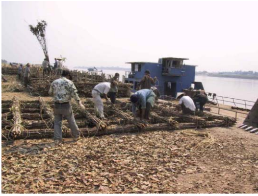
7) Flooring 'Siki-Soda' work
