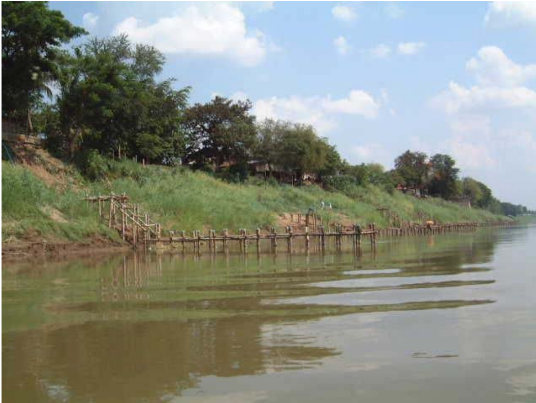
After Construction (May 2003)
