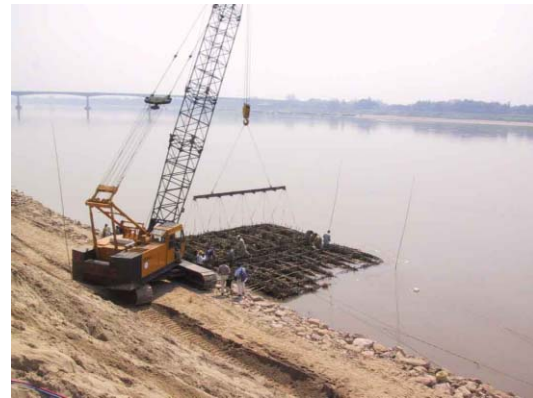
4) Placing Soda mattress at the planned position by Crawler crane
