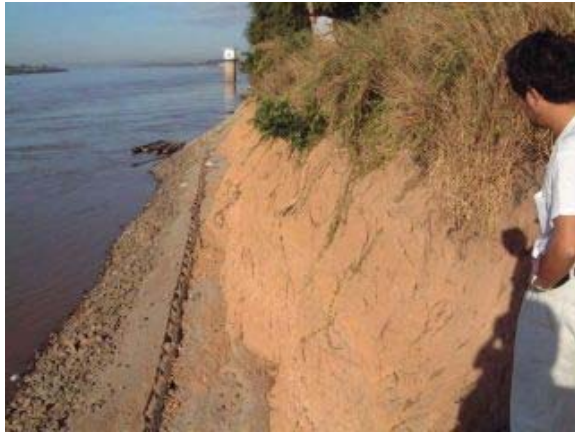
December 15, 2001 <Upstream Side>
