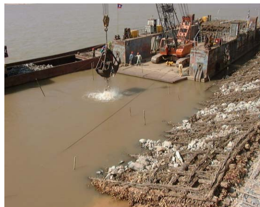
6) Lift and place cobble stone with a crane
