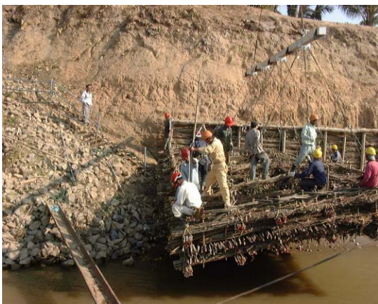
5) Submerge the mattress in the previously designate river position.
