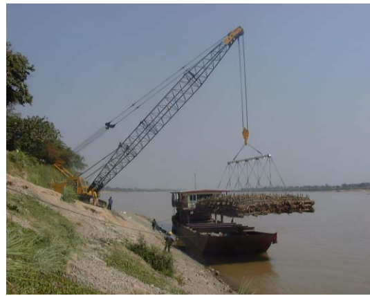
4) Lift and transport the finished mattress using a crane
