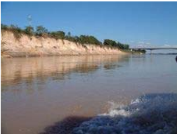
Near Ban Dongphosi Site (around KM1551)
