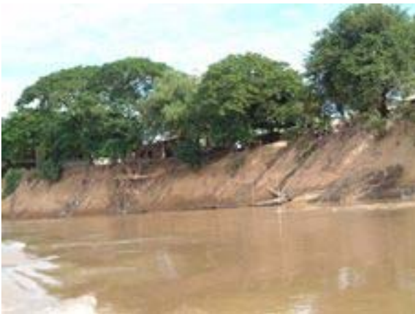
Near Boo Site (around KM1574)
