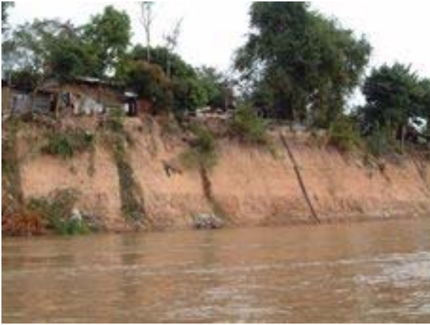
Downstream of Sibounheuang Site (around KM1588)
