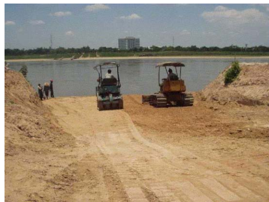
6) Gravel spreading and compaction for the restoration at temporary access road
