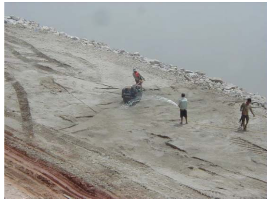
4) Moisture content arrangement by pumping water and compaction by roller
