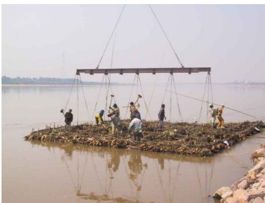
5) Piling of wooden short pile to the final depth
