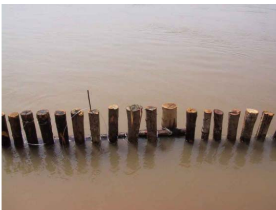
5) Close view of pile arrangement
