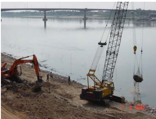
8-1) Putting rubble stones on mattress by wire straw-basket to submerge mattress
