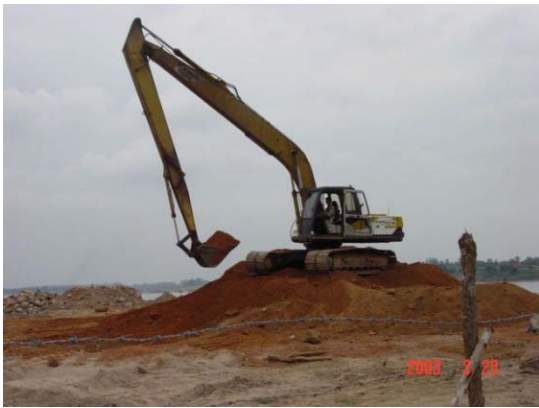
3) Laterite loading by backhoe
