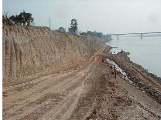
2) Temporary road near riverbed
