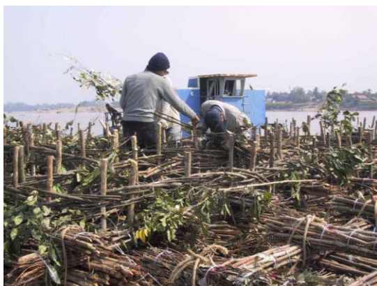
11) Hurdling work by using 'Taisha'
