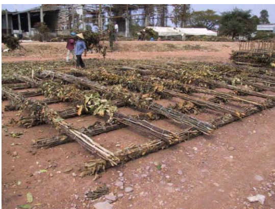
5) Arrangement of lower lattice structure by using 'Rensai'.
