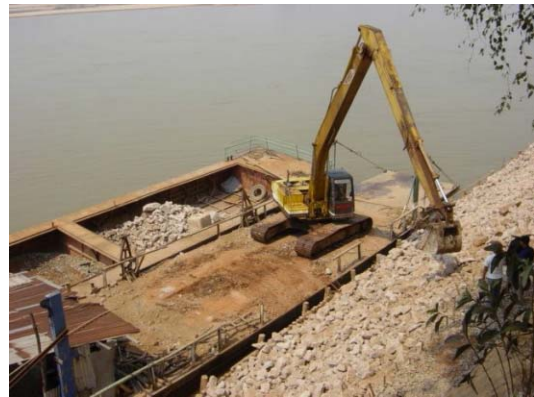
4) Cobble placing by backhoe on barge
