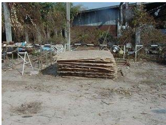
5) Stockpile of bamboo net
