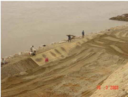
3) Filling of river sand below El. 161.5m
