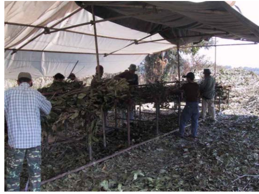
2) Making 'Rensai' (connection beam made of fascine)
