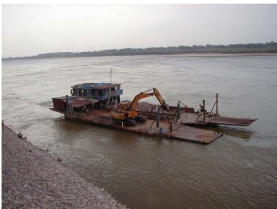
5) Stone placing on Soda mattress from barge
