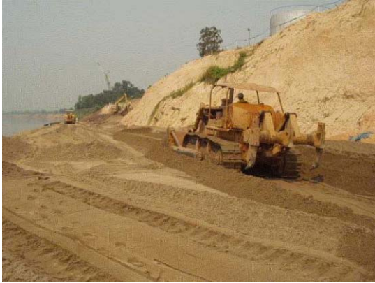
1) Embankment work by bulldozer
