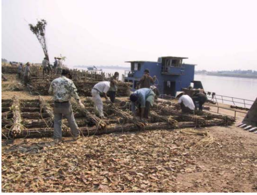
7) Flooring 'Siki-Soda' work
