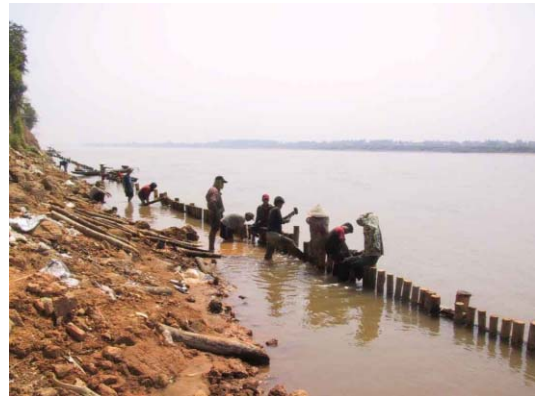
4) Secondary piling work by manpower between primary piles.
