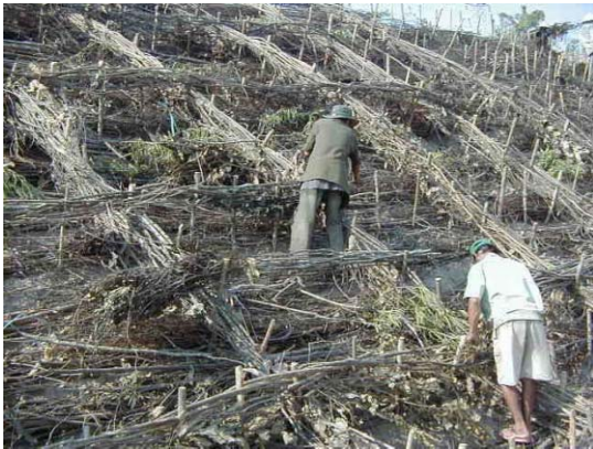
3) Hurdle work using 'Taisya' and Siki-soda placing
