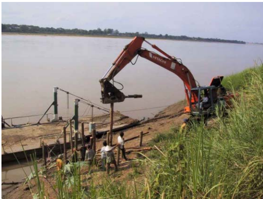
3) Piling work by backhoe (pushing down)
