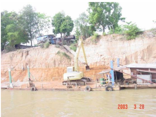
5) Filling and slope compaction by backhoe on barge
