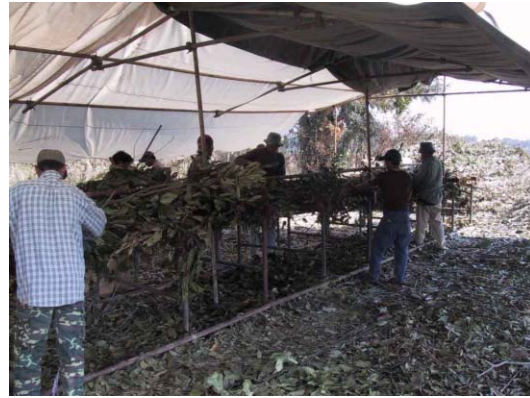
2) Making 'Rensai' (connection beam made of fascine)
