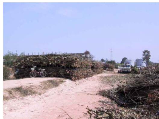
12) Piling-up of completed Soda mattresses
