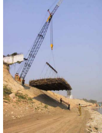
2) Lowering Soda mattress to the bank slope
