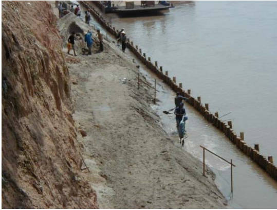
1) Embankment of river sand
