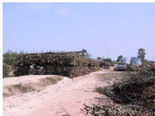
12) Piling-up of completed Soda mattresses
