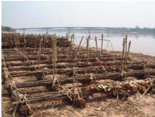
3) Soda Mattress under assembling
