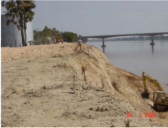
1) Trimming of the slope by backhoe
