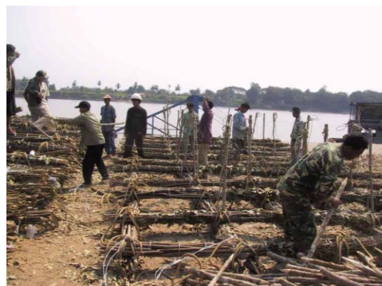
6) Fixing node of Rensai lattice
