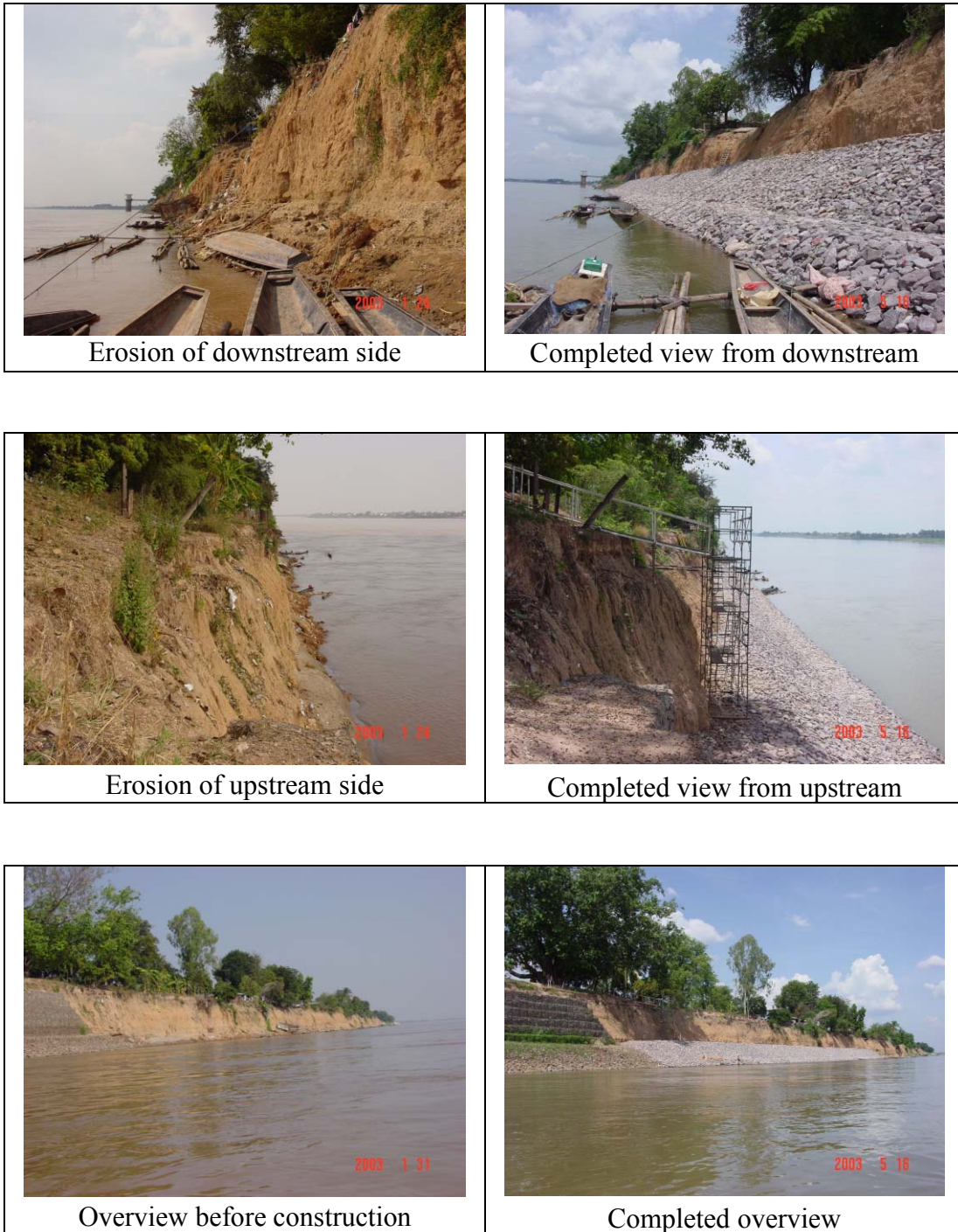
Figure 1.1.2 (3/3) Picture of Pilot Works
