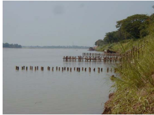
8) View of completed groin works
