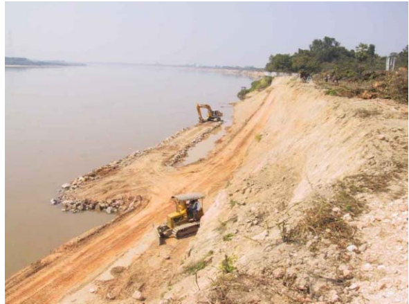
2) Extending the foundation work by Backhoe
