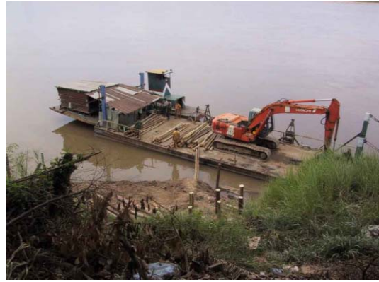
2) Transporting to the wooden piles to the planned location by barge
