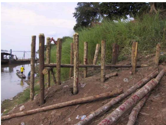
5) Lateral view of piled wooden logs
