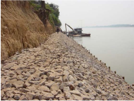
1) View of completed slope protection work
