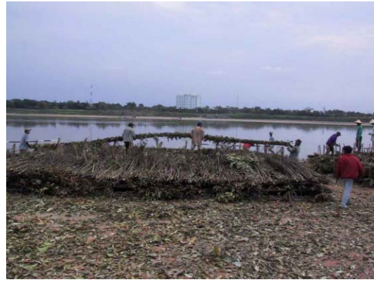
8) Arranging higher lattice beam
