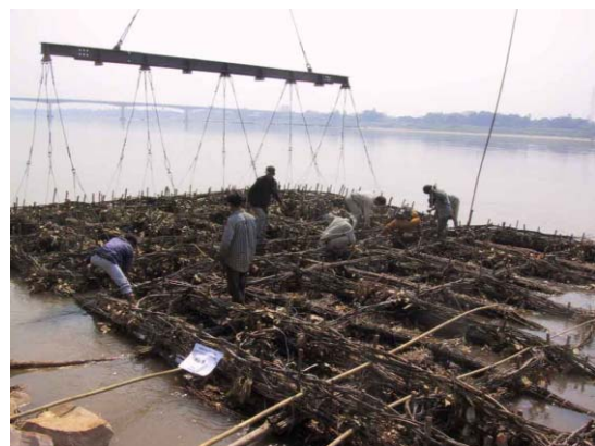
6) Connection of Soda mattress with up-stream one
