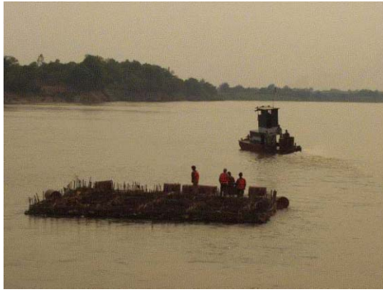
1) Towing floating Soda mattress by boat from Kao Liao stockyard into the site
