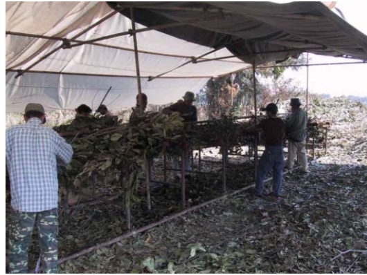
2) Making 'Rensai' (connection beam made of fascine)
