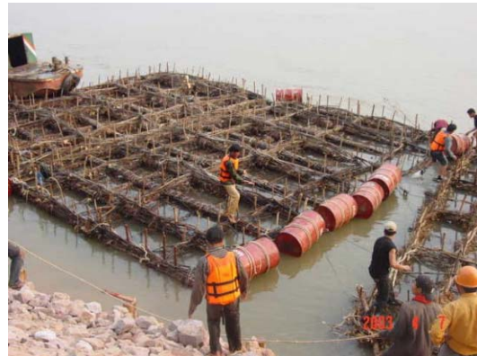
4) Connecting Soda mattresses by manpower
