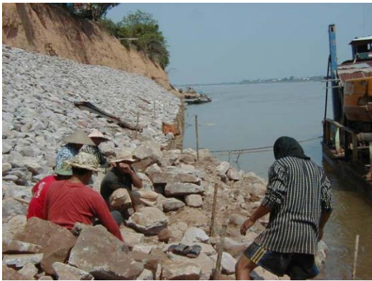
3) Stone placing adjustment by hand around log hurdle work
