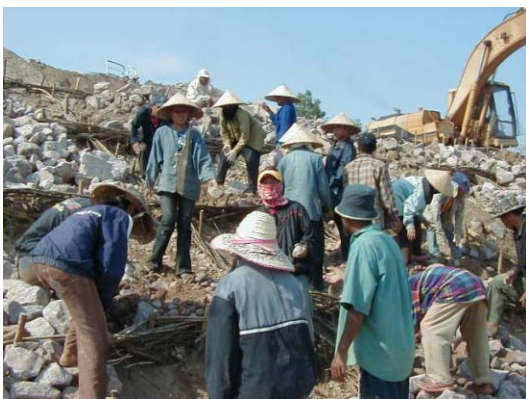
5) Cobble placing by manpower
