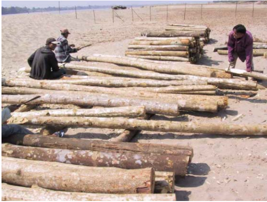
1) Preparation of wooden pile by sharpening tip of log
