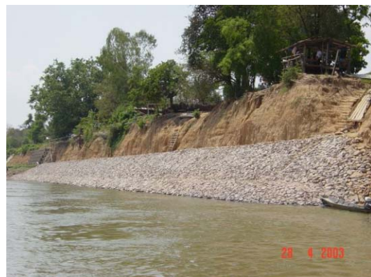
4) Stone placing adjustment by hand under water around the conjunction to Soda mattress
