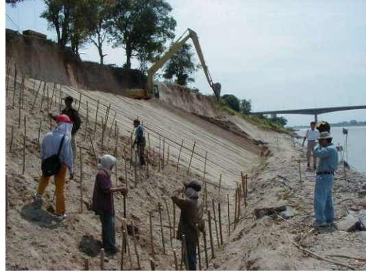
2) Compaction of slope and Kogui piling
