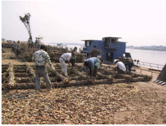
7) Flooring 'Siki-Soda' work
