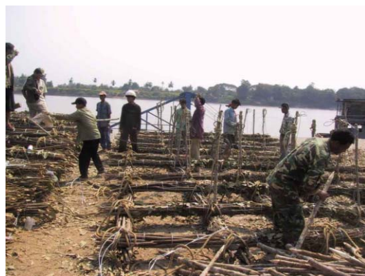
6) Fixing node of Rensai lattice
