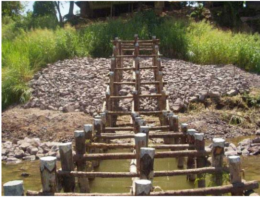
7) Riprap on the slope around connecting piles
