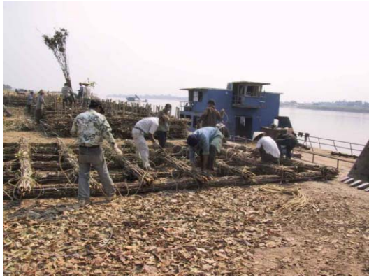
7) Flooring 'Siki-Soda' work
