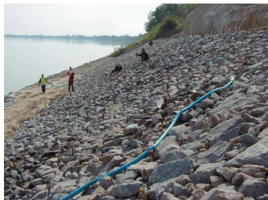
6) Finishing work of slope: Adjusting cobble placing
