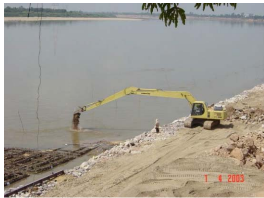
8-2) Putting rubble stones on mattress by backhoe to submerge mattress
