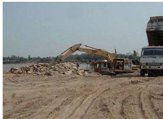
6) Loading into Barge
