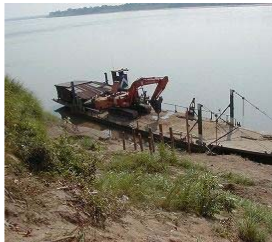
2) Barge and piling
