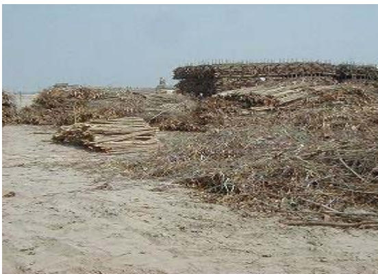
5) Stockyard for fascine, Rensai, Mattress
