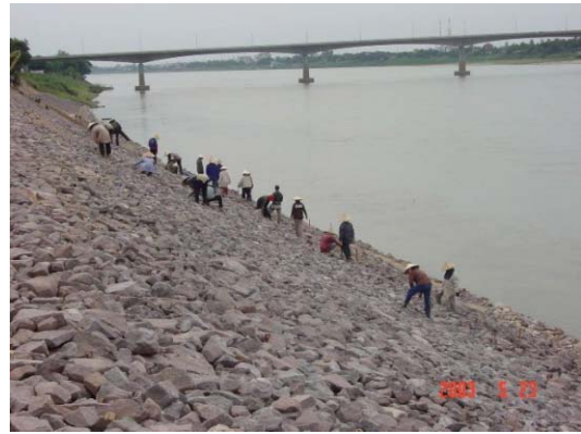
4) Stone arrangement by manpower
