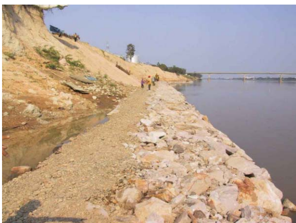
5) Placing gravels behind the rip-rap
