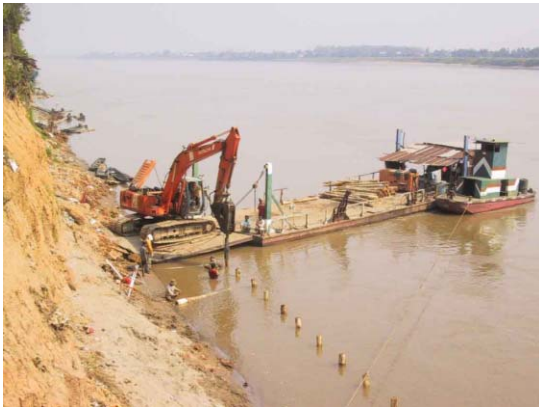
3) Primary piling work by Backhoe mounted on Barge
