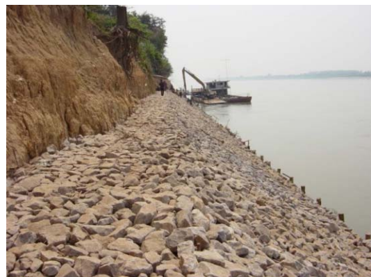
6) Completed cobble stone with willow branch works
