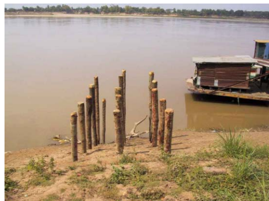
6) Longitudinal view of piled wooden logs
