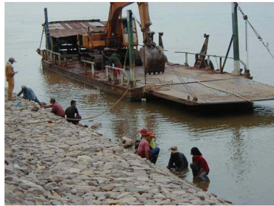
4) Stone placing adjustment by hand under water around the conjunction to Soda mattress
