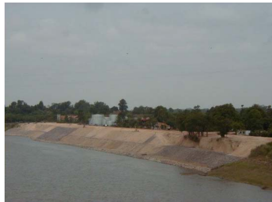
6) Overview of completed pilot works and the stone covering in front of oil tanks
