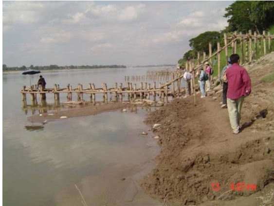
Figure 5.2 Sedimentation between Wooden Pile Dike Groyne Works
