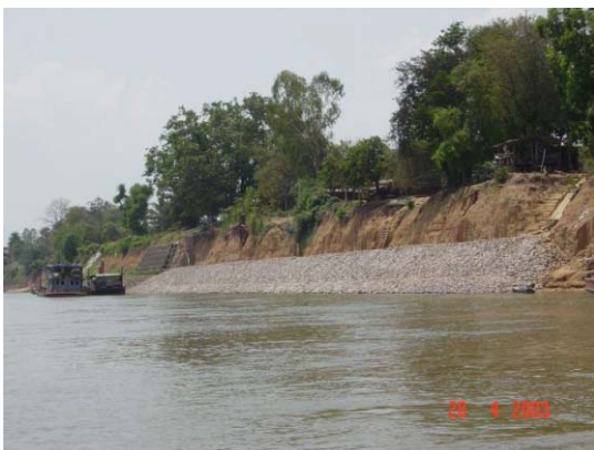
Just after construction (April 2003)
