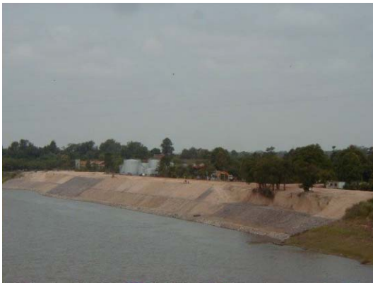
Just after construction (May 2003)
