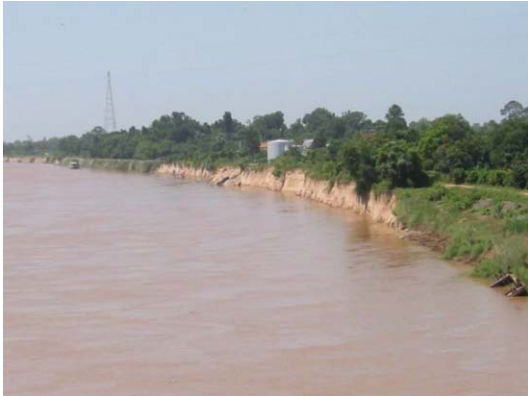
Before construction (October 2002)
