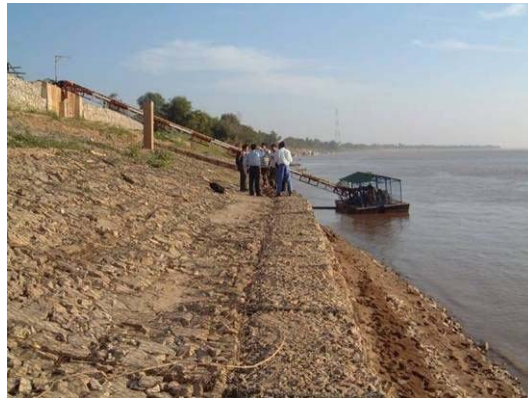
Figure 2.7 Soda Mattress Installed Site at Thakhek - Condition in December 2001-
