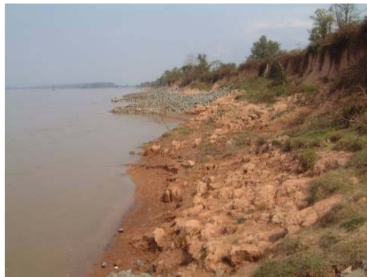
Figure 2.8 On-going Riprap Groin Works in Bokeo Province - Condition in December 2001-
