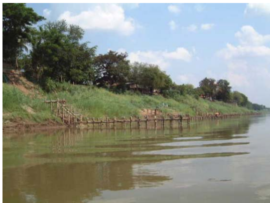
Just after construction (May 2003)
