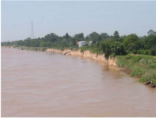
Before construction (October 2002)
