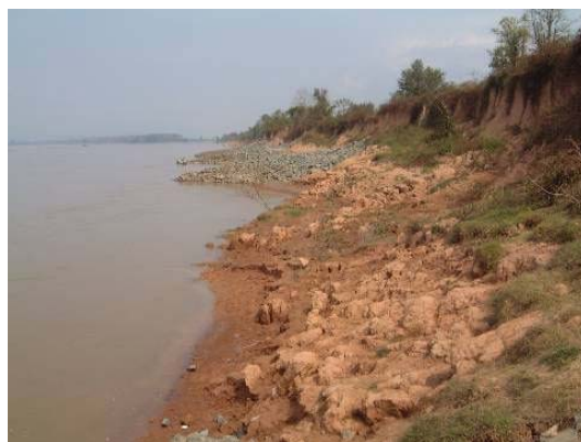
Figure 2.7 On-going Riprap Groin Works in Bokeo Province - Condition in December 2001-
