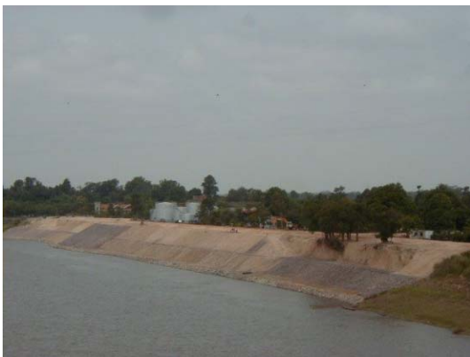
Just after construction (May 2003)
