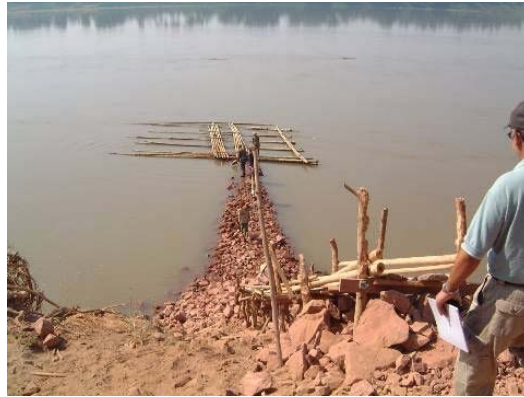
Figure 2.6 Riprap Low Groins at Pakkadan - Condition in February 2002-
