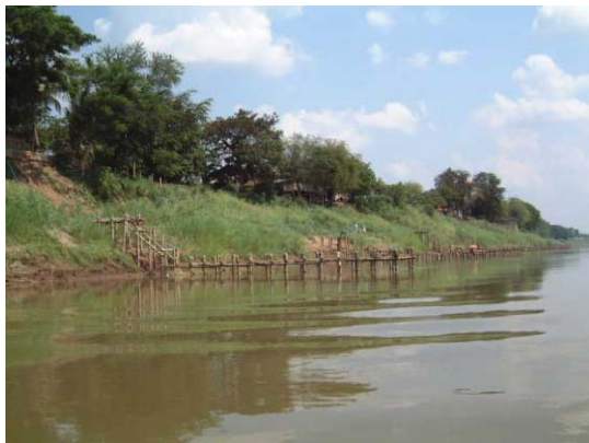
Just after construction (May 2003)
