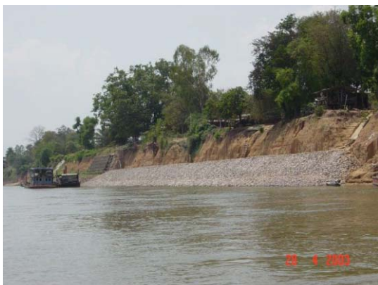
Just after construction (April 2003)
