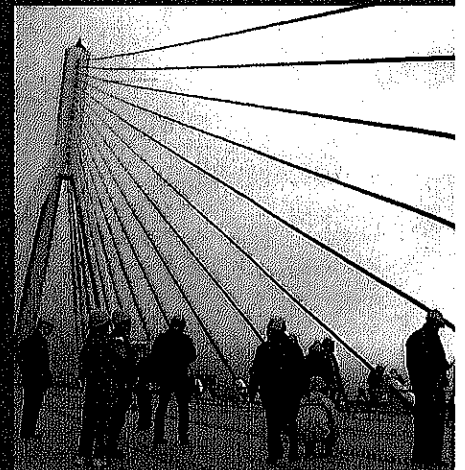
Visit to Mihara Bridge (suspension bridge)
