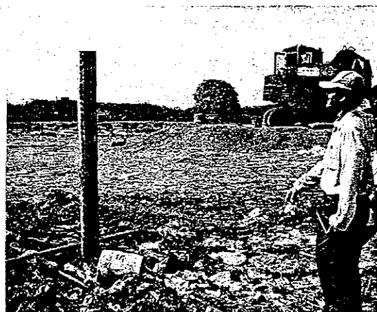
Gas venting pipe
