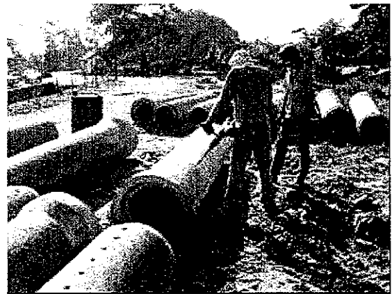
Leachate collection pipe (Main Pipe)
