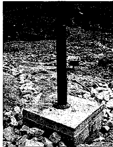
Gas ventilation pipe
