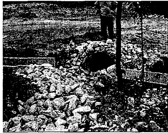
Storm water drainage below access road
