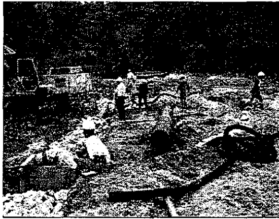
Installation of leachate collection pipe
