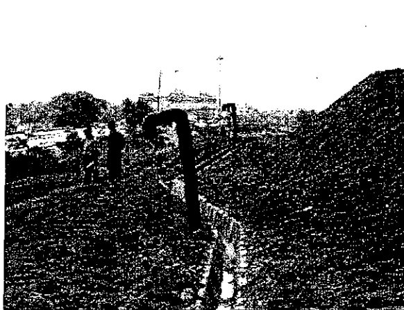
Gas ventilation pipe
