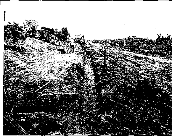
Installation of leachate pipe/drain
