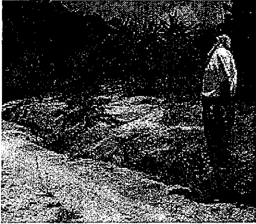
Plate A9-1 Surface Erosion
