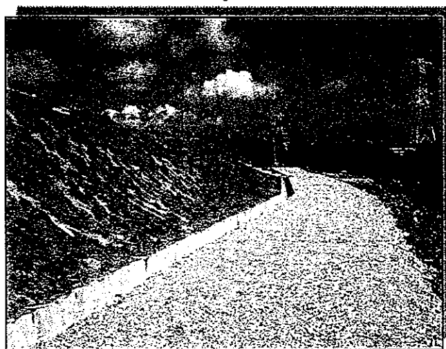
After PP (Improved slope, drainage, leachate collection (not visible) and access road)
