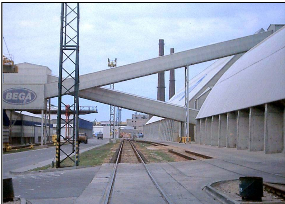
Photo III.6.3-9 Covered conveyors at the Bega Terminal
