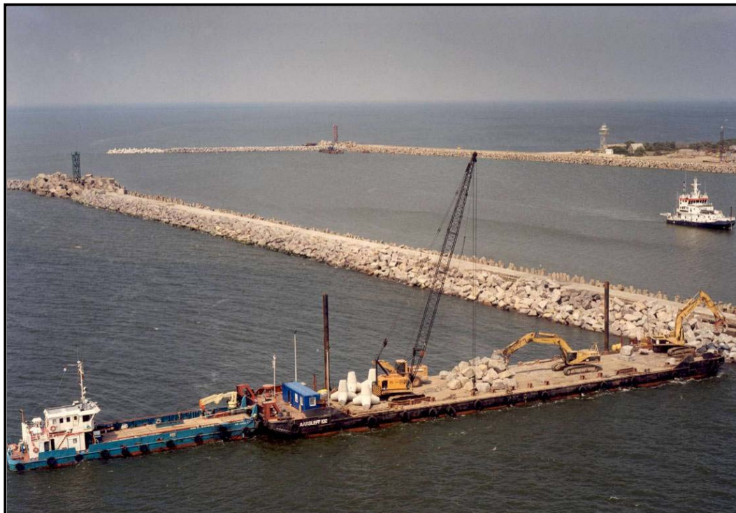
Photo III.6.3-3 Operation to replenish rock protection on the southern breakwater
