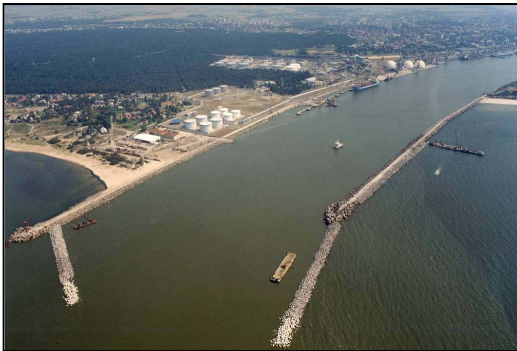
Photo III.6.5-8 Landscape of the northern port showing the Nafta and Klasco Terminals and Giruliai Forest and Melnrage on the left
