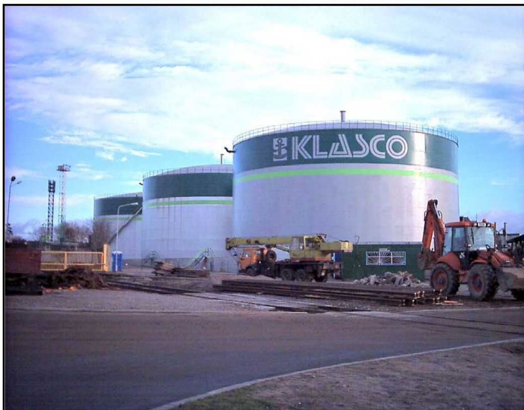
Photo III.6.3-7 Storage tanks at Klasco Terminal
