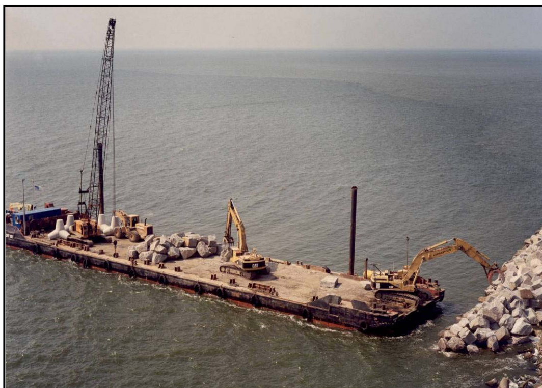
Photo III.6.3-2 Likely construction method for breakwaters and revetments
