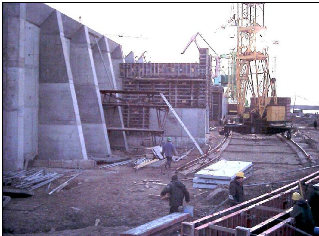
Photo III.6.3-5 Warehouse under construction at Klasco Terminal in December 2003
