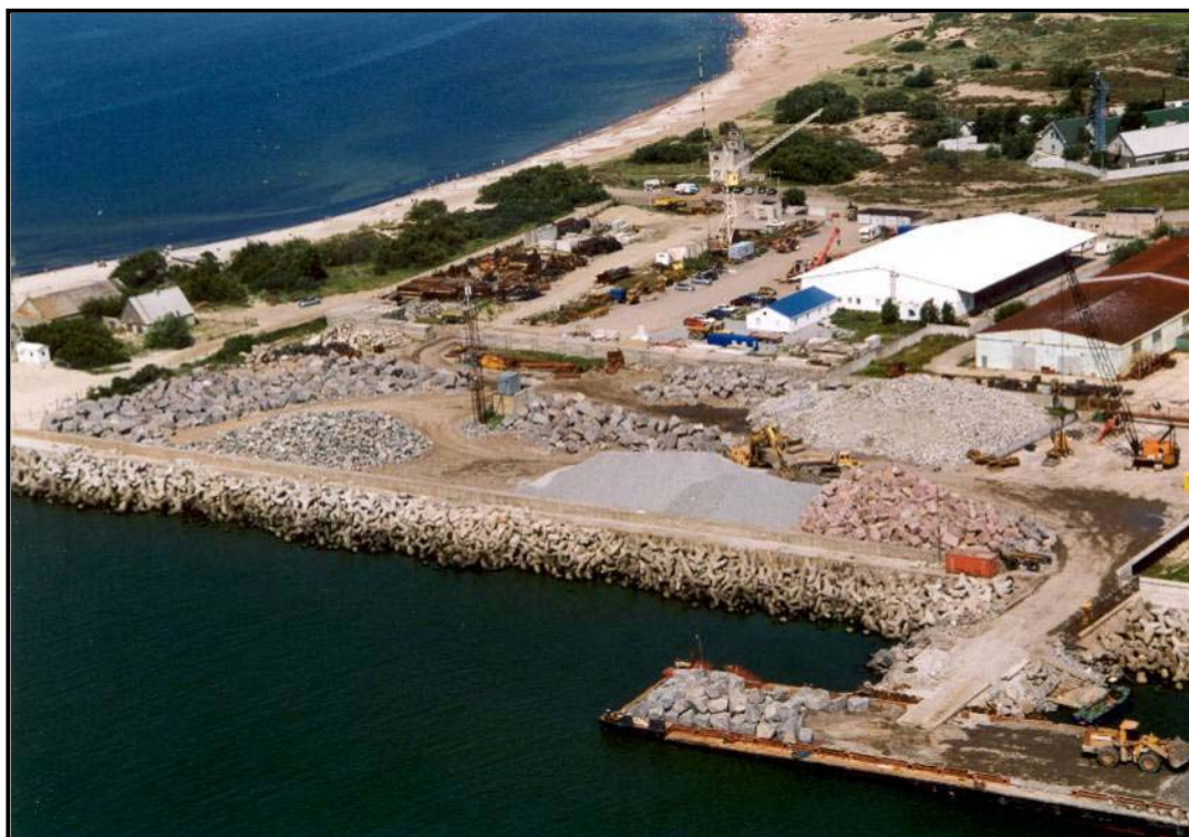
Photo III.6.3-1 On-land construction site for breakwater extension project (2002)
