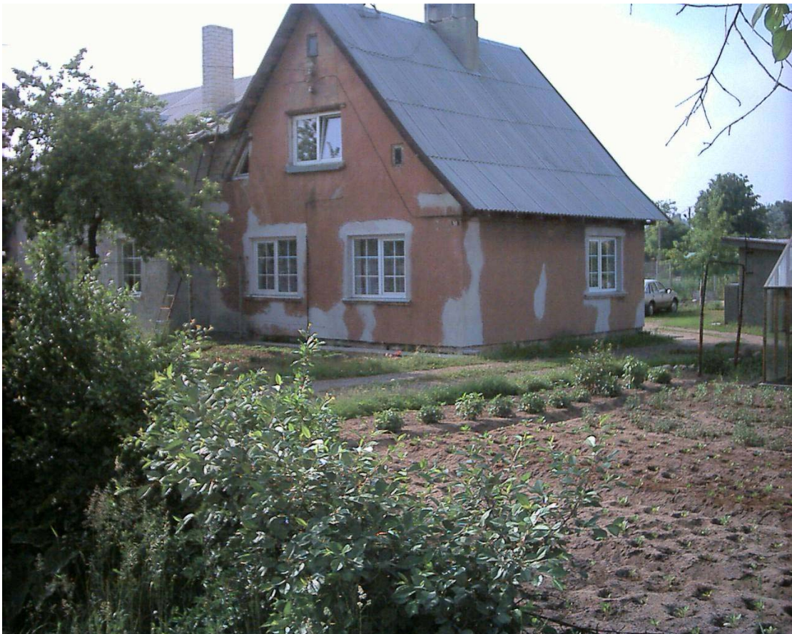
Photo III.5.3-3 Potential Port Development Site C: Reserved Port Territory around the Smeltale River, east of the Fishing Harbour
