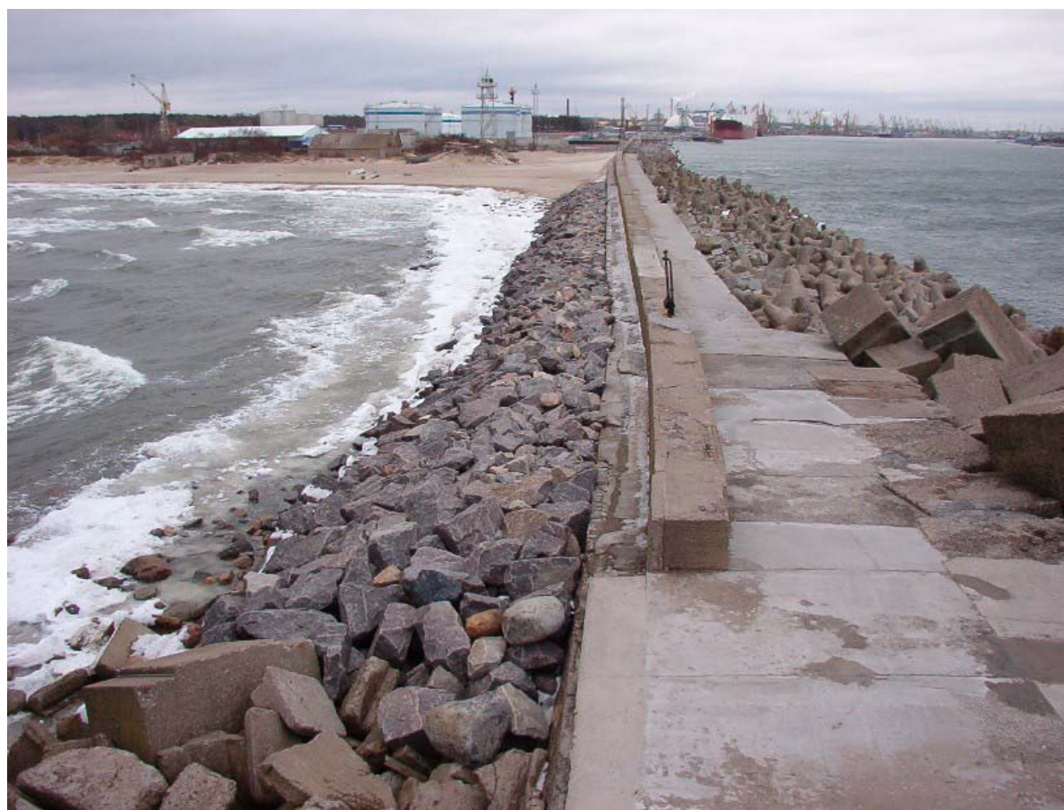
Photo III.5.2-8 Breakwaters at the mouth of the Port Channel
