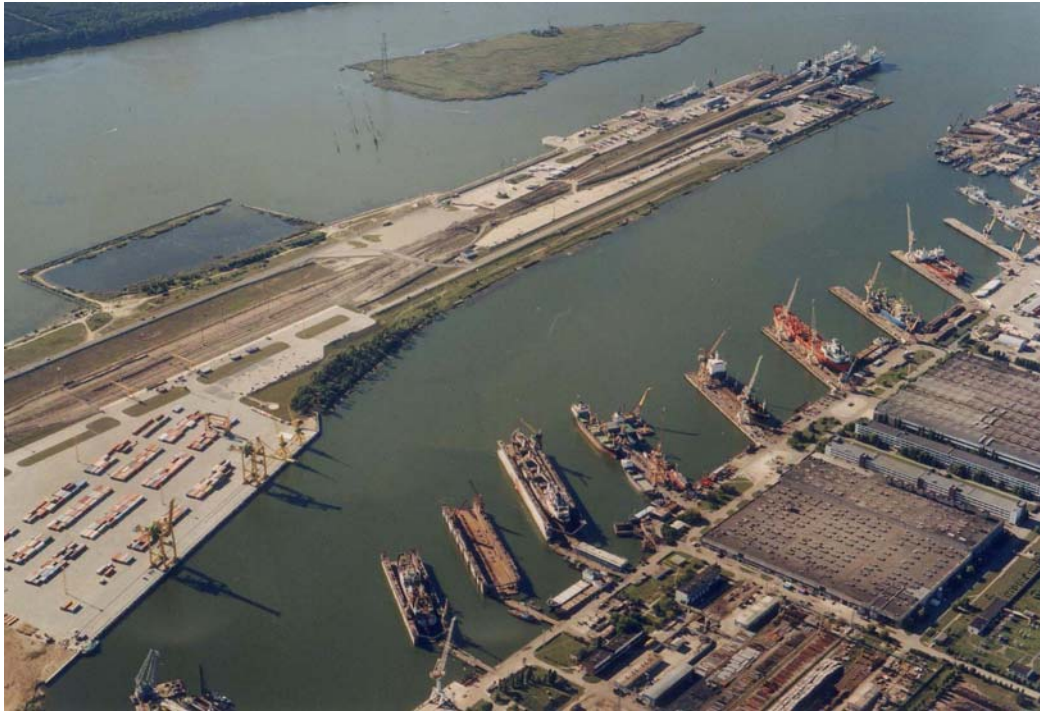
Photo I.2.2-8 Western Ship Repair Yard
