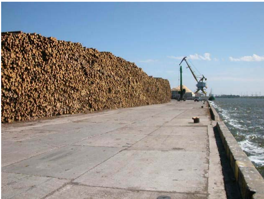
Photo I.2.2-9 View of Berth No.118
