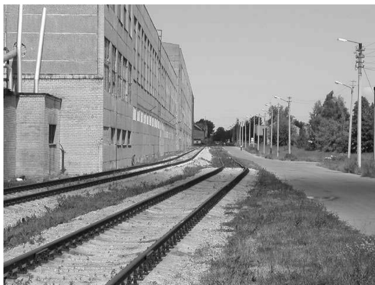
Photo I.2.5-7 Double Track in front of BEGA
