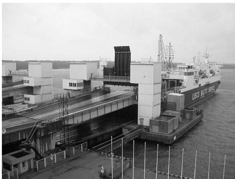
Photo I.2.5-12 International Ferry Terminal
