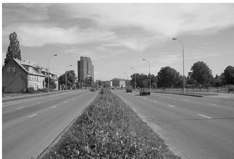
Photo I.2.6-5 Minijos Street with Six-lane
