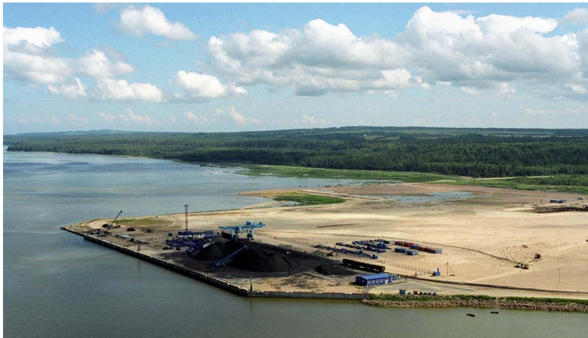
Photo I.1.1-4 Ust Luga Coal Terminal, June 2003 (Main development area beyond)
