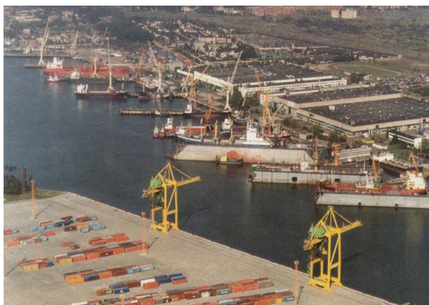
Photo 2.3 Container Terminal of EUROGATE (KLASCO)
