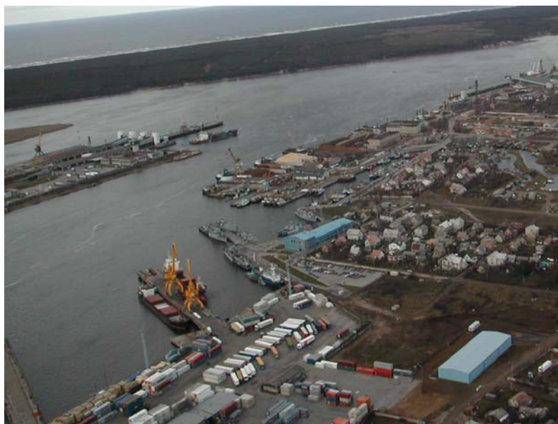
Photo 2.6 Facility Layout of Klaipedos Terminals
