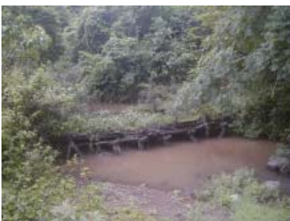
Photo 8.5 Weir put together by wood
