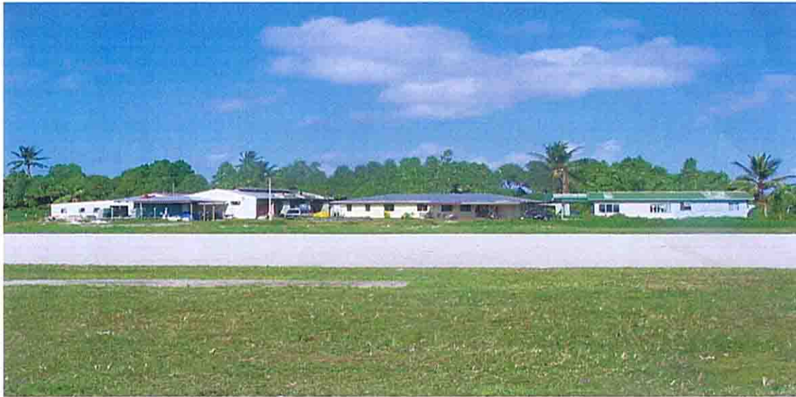
Photo.1: Existing Power Plant Complex
