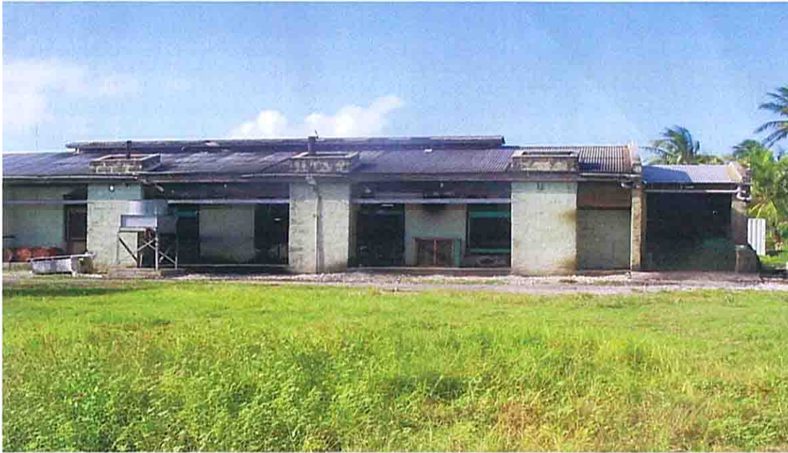
Photo.3: Existing Power House
