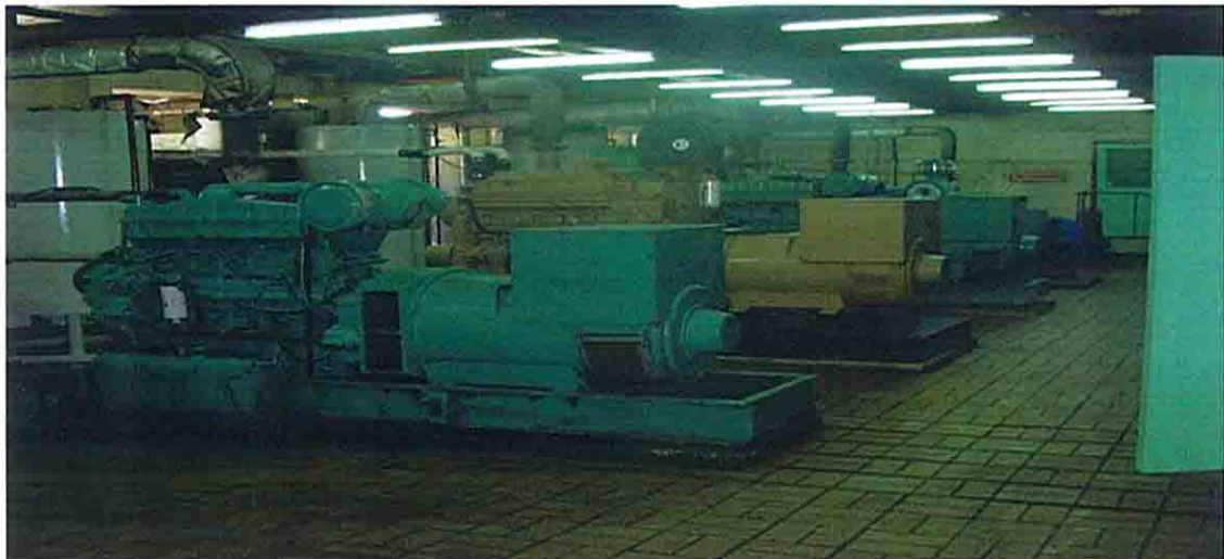
Photo.2: Existing Power Generators
