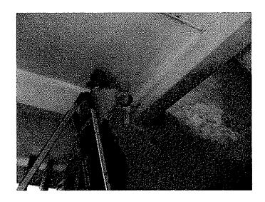
Stair No2 E-2 Chipping Beam for testing
