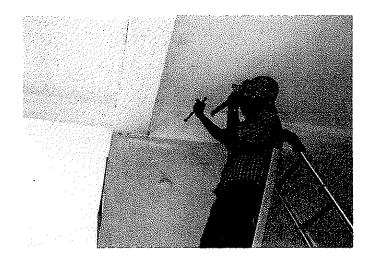
Stair No1 E-2 Chipping Beam for testing
