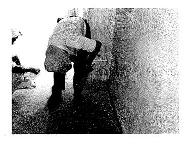
Stair No2 E-1 Chipping Column for testing
