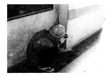
Stair No1 E-1 Chipping Column for testing
