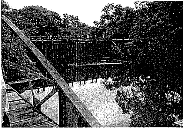
Kunchukulam Head Sluice Source of Giants Tank
