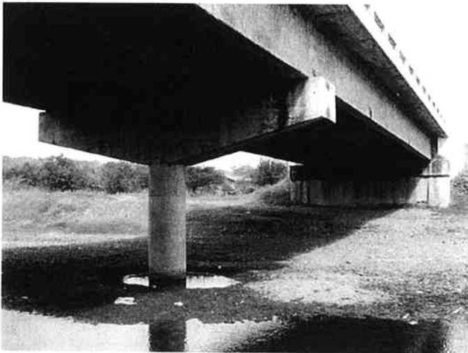
Pier column and its foundation
