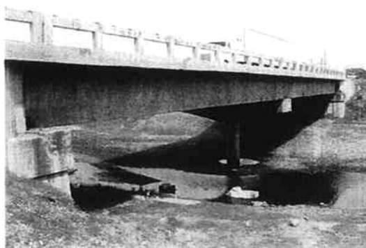
Side View from downstream
