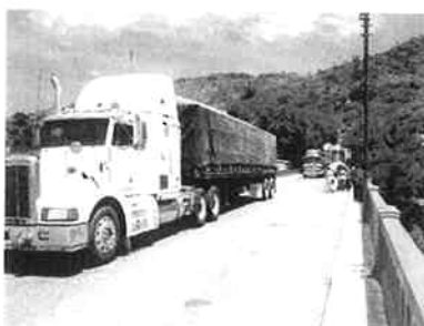
Vibration check on Puente Amatillo
