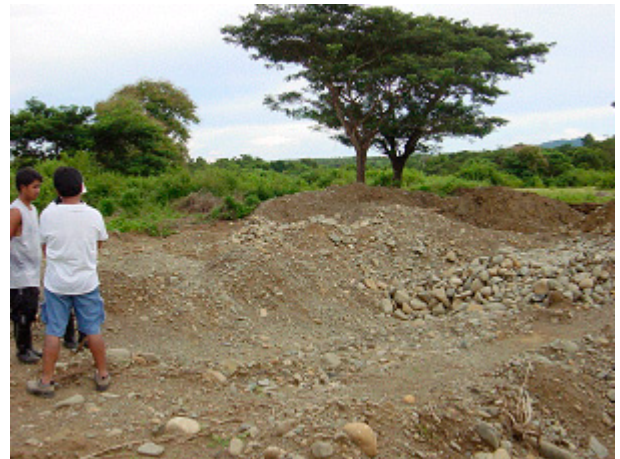
Picture A.5.7 Condition of Powerhouse Candidate Site for Iwahig 2 and 3
