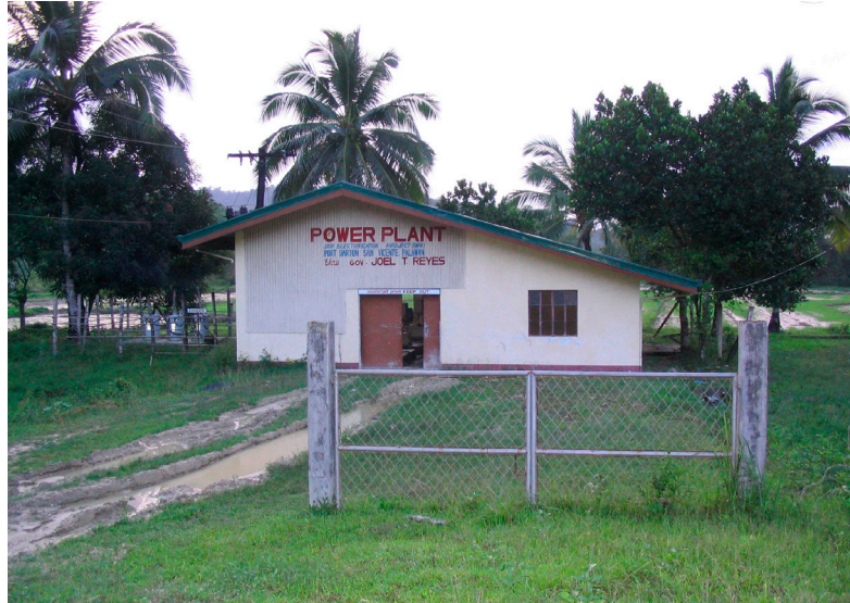
Figure 3.2.4 Port Barton Power Plant
