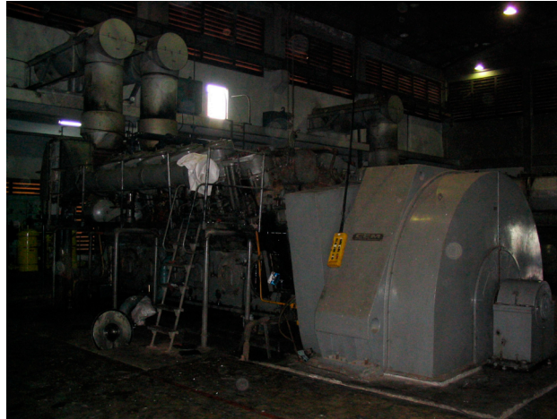
Figure 3.3.8 No. 2 Unit Under Corrective Maintenance
