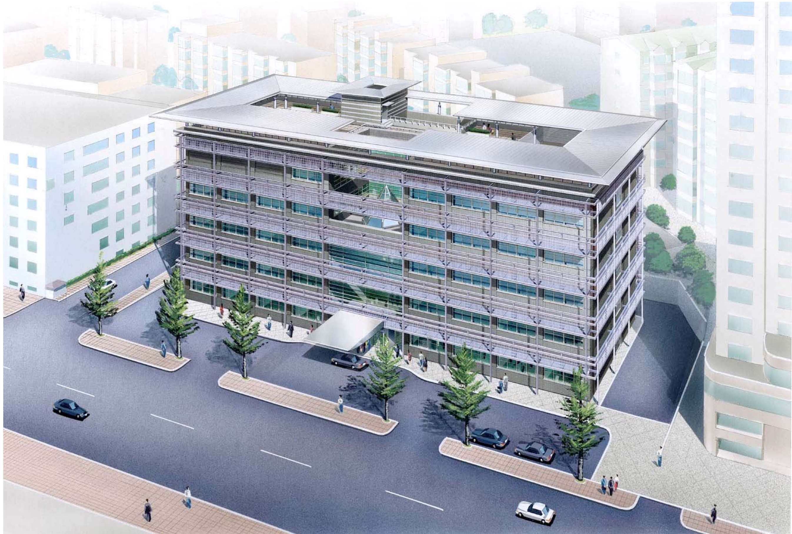
THE PROJECT FOR CONSTRUCTION OF THE CHINA-JAPAN FRIENDSHIP DALIAN CENTER FOR HUMAN RESOURCES DEVELOPMENT
