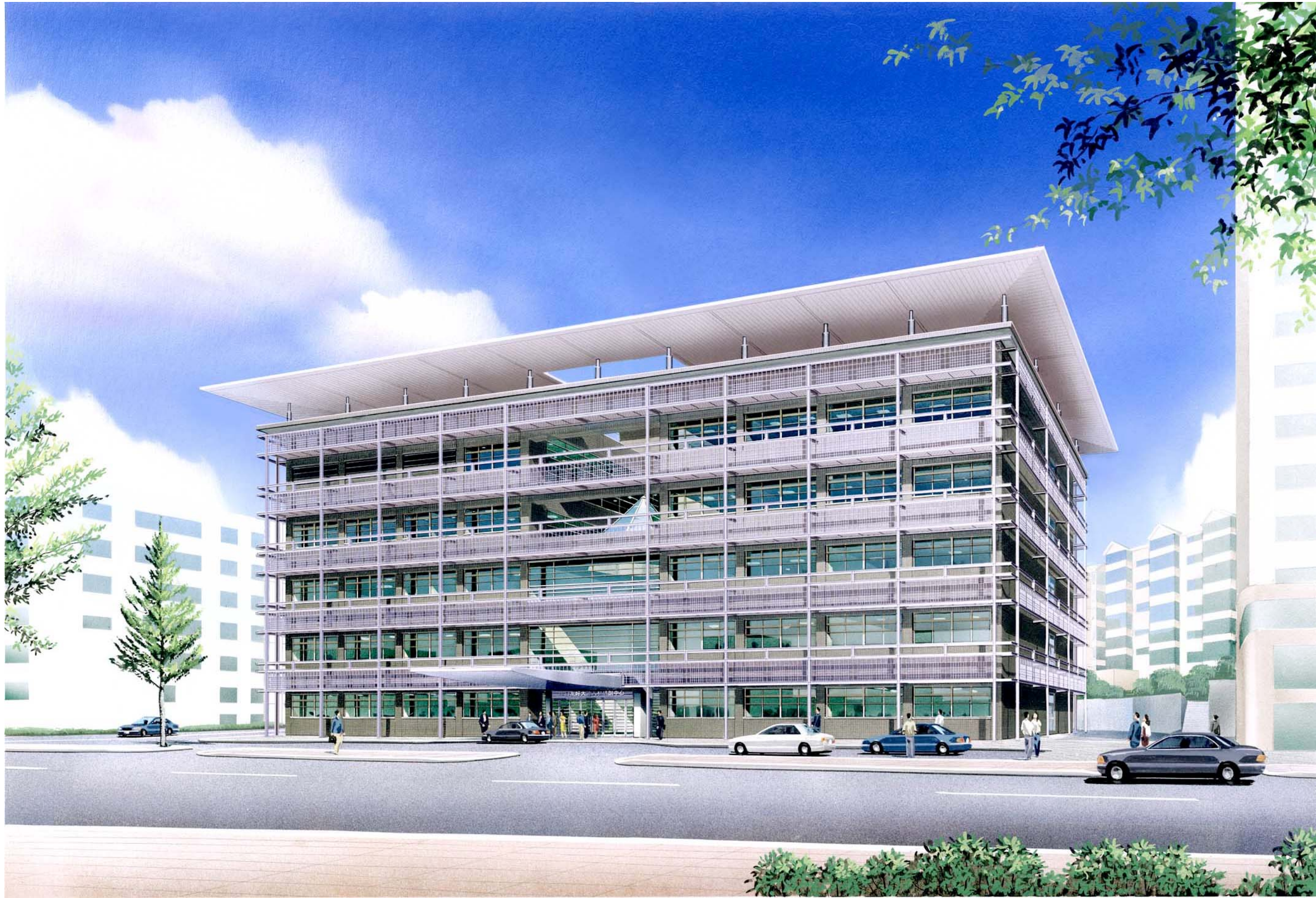
THE PROJECT FOR CONSTRUCTION OF THE CHINA-JAPAN FRIENDSHIP DALIAN CENTER FOR HUMAN RESOURCES DEVELOPMENT
