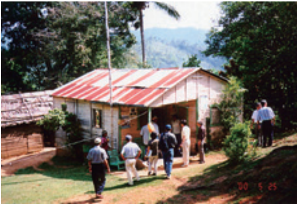
The “Project for Agricultural Development on Sloped Terrains” in the Dominican Republic. Farmhouse on Sloped Terrains.
