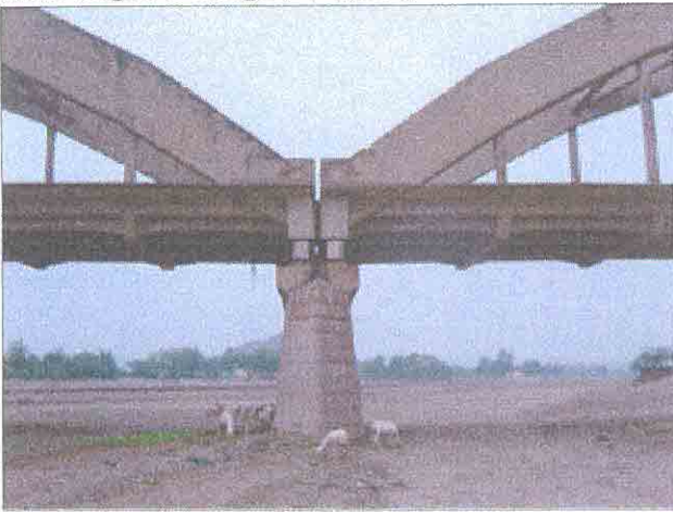
No.4 Dogali 1 Bridge / P1(Mov)
