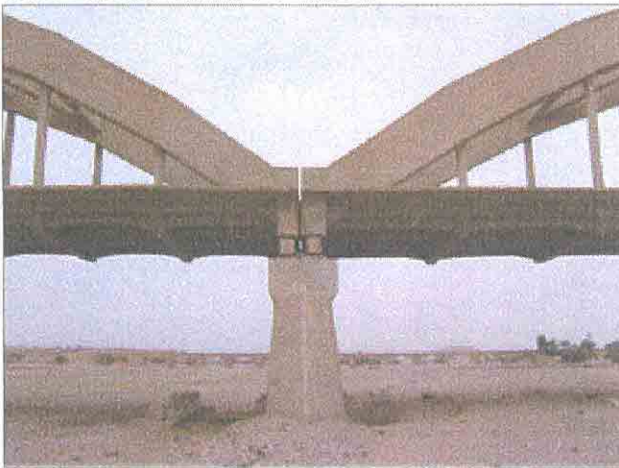
No.6 Emculu Bridge / P1(Mov)
