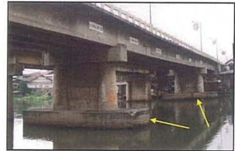
Photo 24.1.1-3 Enlarge pile cap and additional piles (not seen on picture)
