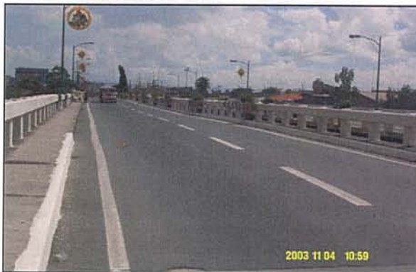
Photo 24.1.3-1 Road / Deck Level Inspection
