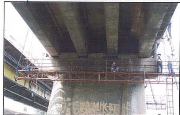
Photo 24.1.3-2 Below Deck Level Inspection
