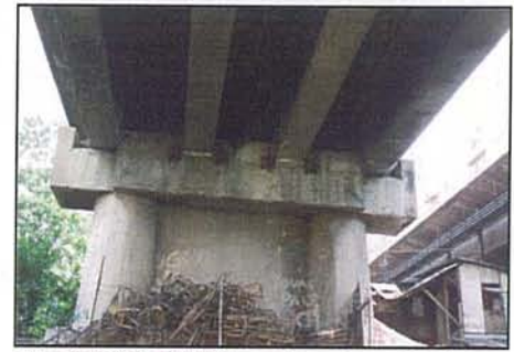
Photo 24.1.1-2 Shear keys on all piers and vertical cable restrainers on Pier 1
