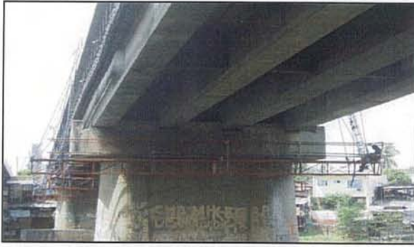
Photo 24.1.3-3 Use of Gondola on below deck inspection
