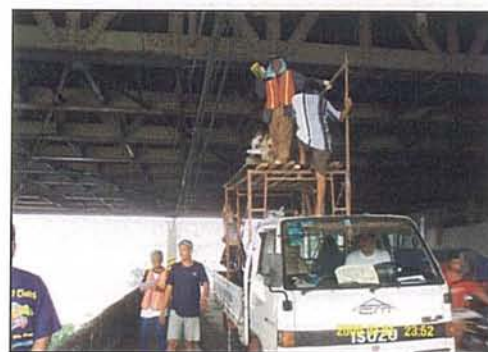
Photo 23.1.3-5 Truck Mounted Scaffolding
