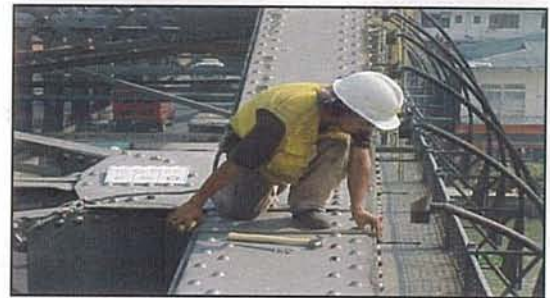
Photo 21.3-7 Measurement of Top Chord Members
