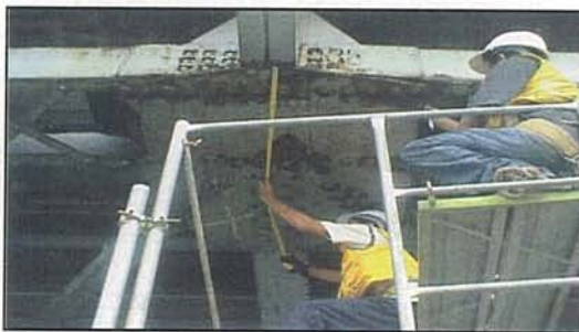
Photo 21.3-8 Measurement of Deck Gusset
