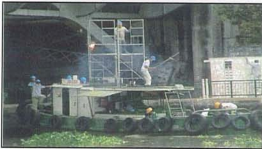
Photo 21.3-6 Tugboat with mounted Scaffolds and Working Platforms
