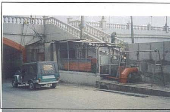
Photo 20.5-1 Photograph showing that there are no Encroachments at the Site of the Jones Bridge
