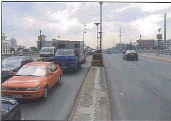
Photo 20.1.3-1 Road / Deck Level Inspection
