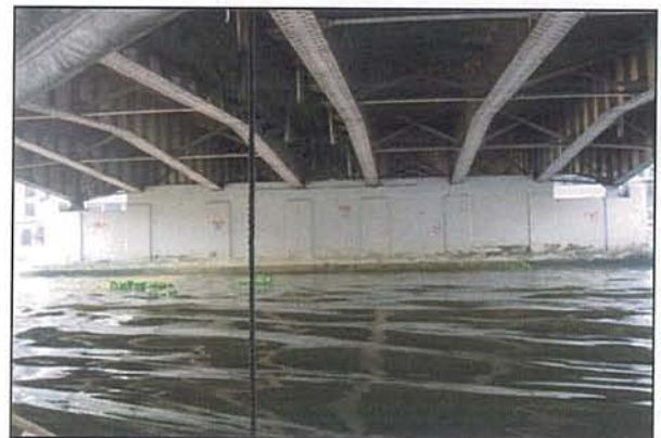
Photo 20.1.3-2 Below Deck Level – Bottom Soffit of Steel Girders and Sway Bracings
