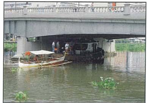
Photo 20.1.3-3 Tugboat with Scaffoldings, and Canoe - Equipment used in Below Deck Inspection
