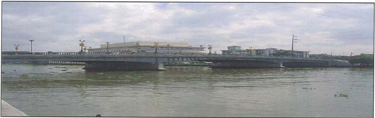
Photo 20.1.1-1 Panoramic View of Jones Bridge
