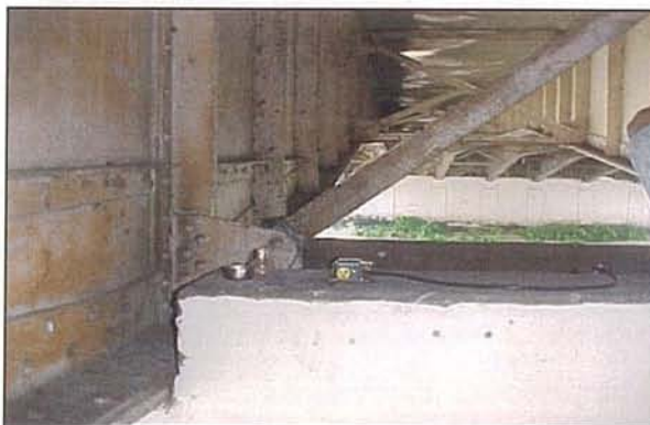
Photo 20.1.3-4 Sensor Location B, off center on top of Pier P2
