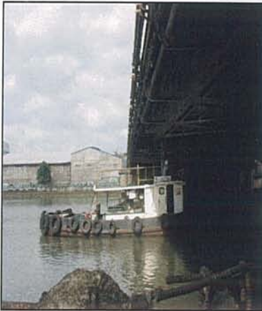
Photo 13.3.1-8 Measurement of Below Deck Level Using Tugboat
