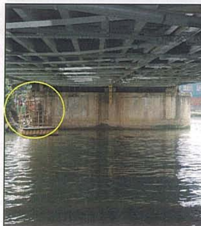
Photo 13.3.1-9 Measurement of Below Deck Level Using Pontoon
