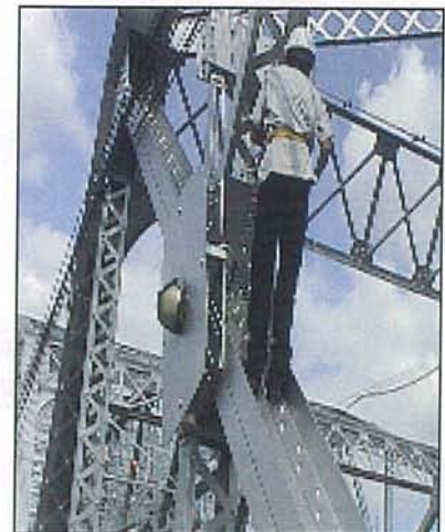
Photo 13.3.1-7 Measurement of Mid Height Gusset Plates and Truss Members
