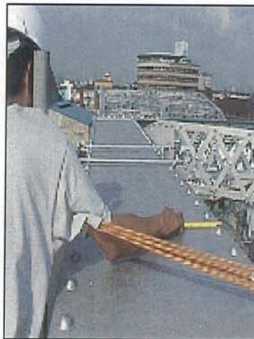
Photo 13.3.1-6 Measurement of Top Chord Member
