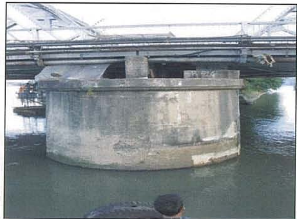
Photo 13.3.1-4 Substructures and Bearings - Pier Shown (Looking East)
