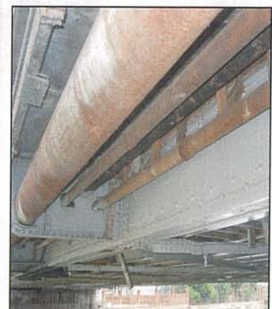
Photo 13.3.1-10 Miscellaneous structures (Pipes)
