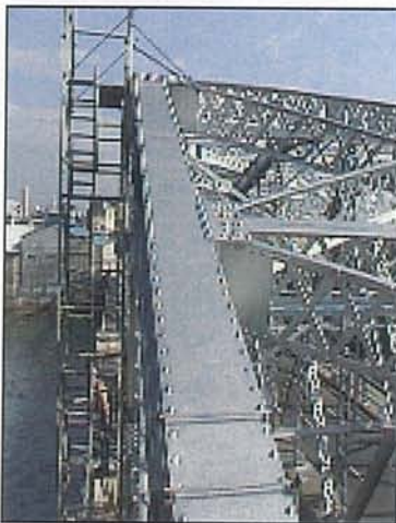
Photo 13.3.1-5 Use of Scaffolding at Main Truss
