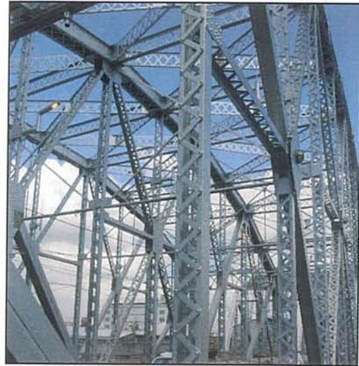
Photo 13.3.1-2 Above Deck Level - Main/Truss Members, Gusset Plates, and Sway Braces
