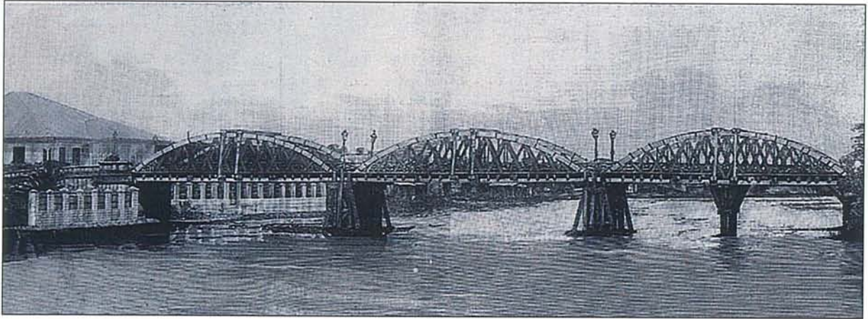
Figure 13.1.3-2 Ayala Bridge After Repair Works (Added Pier at the Center of Right Span) in 1890 (South Span Side)
