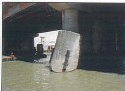
Picture 11.2.1-1 RC Fender Type (C-5 Bridge)
