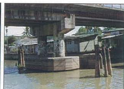
Picture 11.2.1-3 Expanded Footing and Wooden Fender Type
