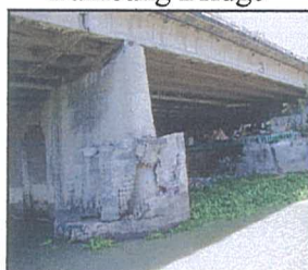
RC Fender Type Connected with Expanded Footing (Guadalupe Bridge)
