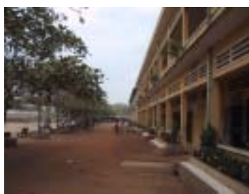
Two-Story Classroom Building (granted by a Norwegian NGO)
