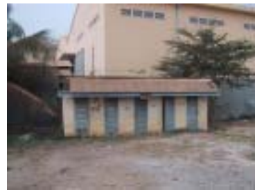
Toilet Facilities for Pupils No longer used. To be demolished.
