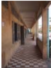
Open Corridor in Three-Story Classroom Building
