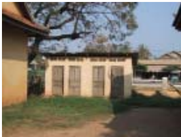
Toilet Facilities for Pupils
