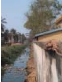
Drainage Conduit Drainage main pipe will be installed parallel to the existing conduit shown in the picture.
