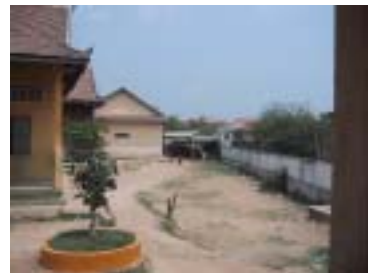
Construction Site for Project Toilet Facilities
