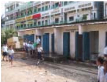
Toilet Facilities for Pupils
