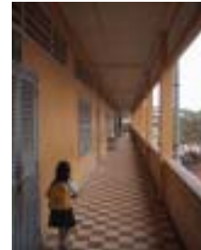
Open Corridor of Two-Story Classroom Building
