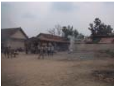
Existing Canteen Building Granted by a French NGO. Required to be demolished as it hinders the construction of project classroom building
