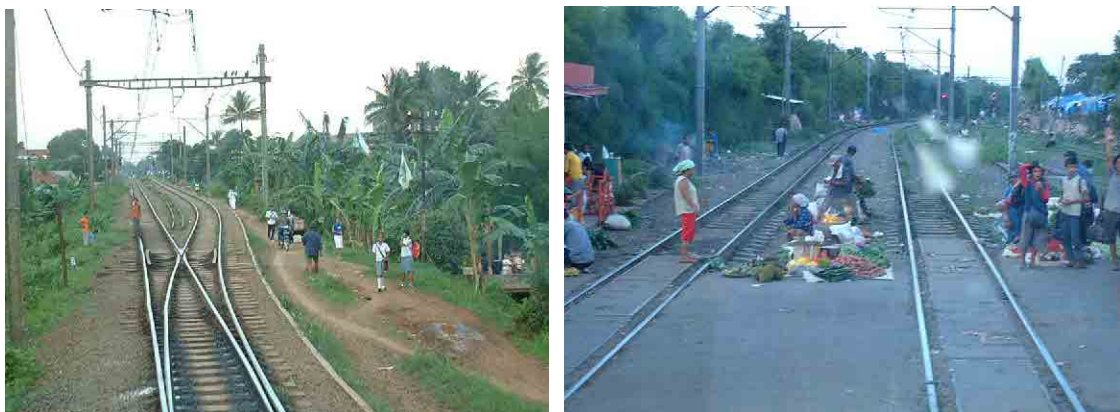
Figure 4.13.2 Present Use of Railway Track
