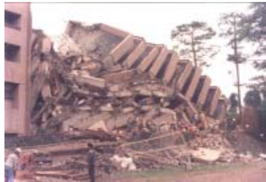
Hyatt Hotel, Baguio City, 16 July 1990 Luzon Earthquake
