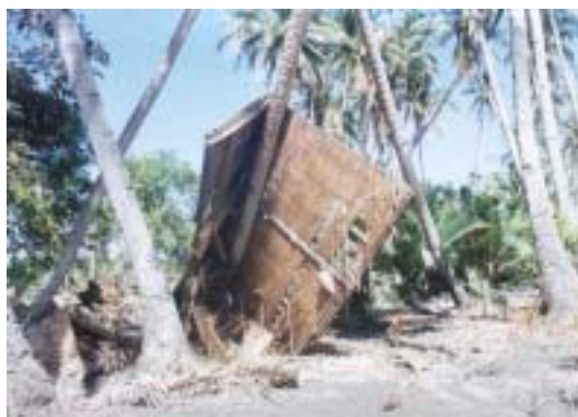
Brgy. Malaylay, Baco, Oriental Mindoro, 15 Nov. 1994 Mindoro Earthquake
