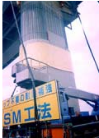
Figure 19.2.9 Example of RC Jacketing Method
