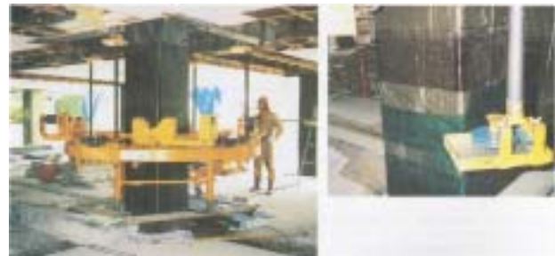
Figure 19.2.11 Example of Fiber Jacketing Method
