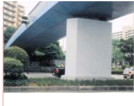
Figure 19.2.10 Example of Steel Jacketing Method
