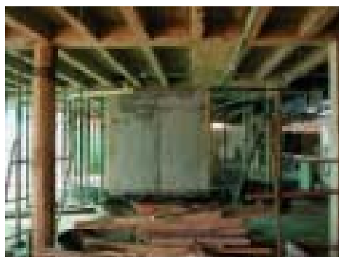
Photo 1 Additional Concrete Wall Installed at the Ground Floor
