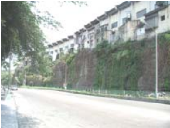
Picture-3 Multiple Residential Housing on Top of Slope
