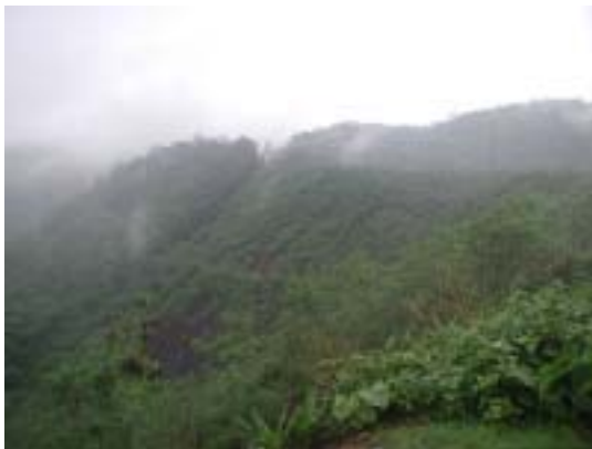
Picture 3. Dike view from crest
