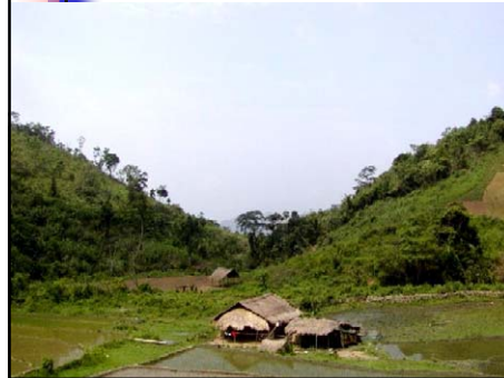
Dan site view from upstream
