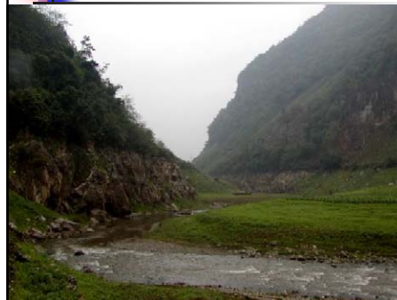
Appeared rocks at the dam site
